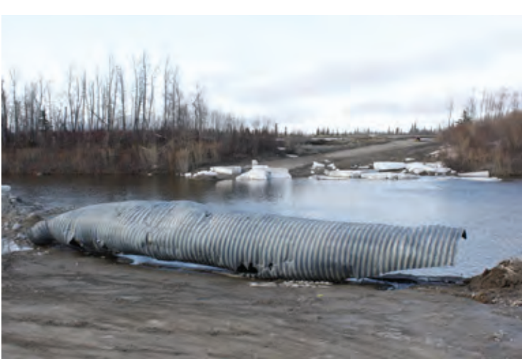
Fig. 22 - Leftover metal from the bridge to the sewage lagoon. The road continues on in the distance across the creek.
