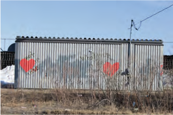
Fig. 21 - Water treatment facility located in the north east corner of the dike.
