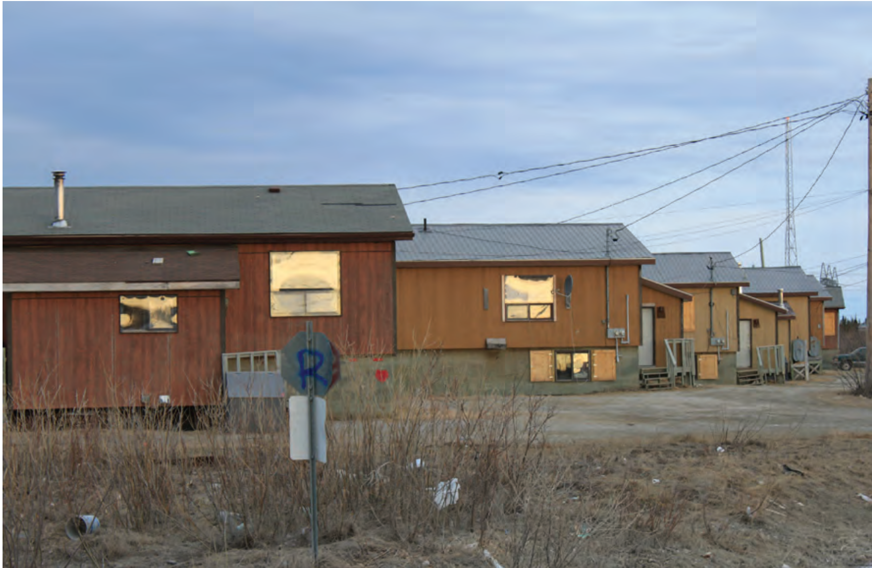
Fig. 31 - One row of the teacher's housing. The reflectivity of the windows is caused by the sheets of plexi-glass that are screwed overtop the exterior frame in an effort to protect the windows from rocks and other objects thrown by kids. This is a huge fire safety issue.
