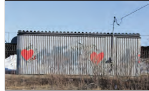
Fig. a239 - Water intake facility
