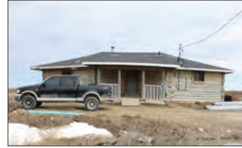
Fig. a95 - House (the only house built out of logs in the community)
