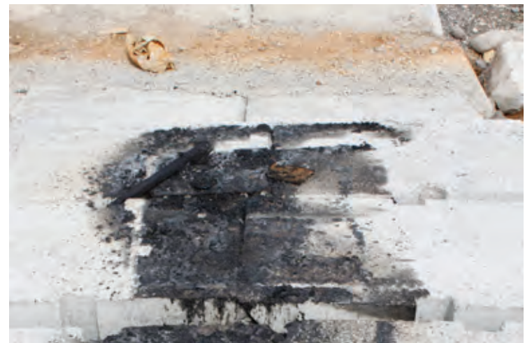
Fig. 72 - Charred remains left by an unknown source on the concrete blocks lining the edge of the dike.
