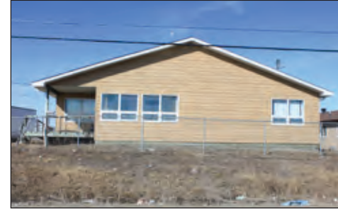
Fig. a203 - Nursing station building
