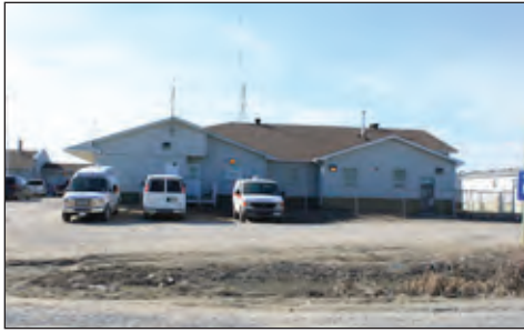
Fig. a205 - Nursing station buildings
