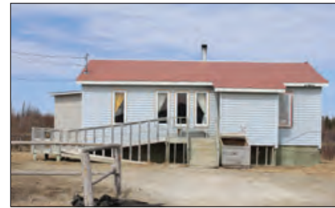
Fig. a132 - House with accessible ramp
