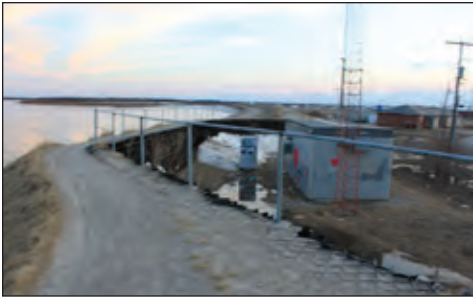
Fig. a242 - Water intake facility
