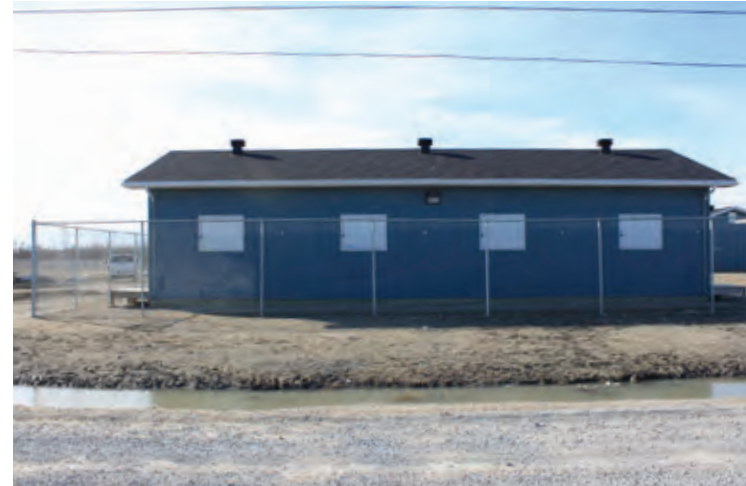
Fig. 16 - One of the portable style school rooms that make up the St. Andrew's elementary school. These buildings are surrounded by chain link fences with basketball nets in between each classroom unit.
