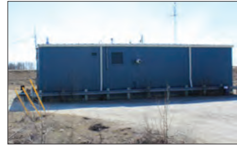
Fig. a262 - Municipal building
