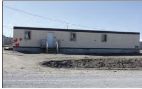
Fig. a29- Offices
