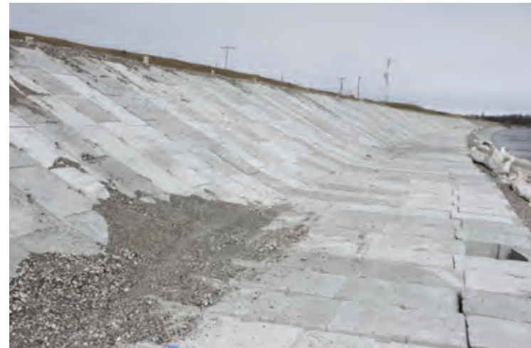
Fig. 28 - Concrete blocks, installed in 2010, protect the dike from yearly erosion. This image shows the dike after its first winter. Many blocks have shifted but the overall system seems to be functioning as intended.
