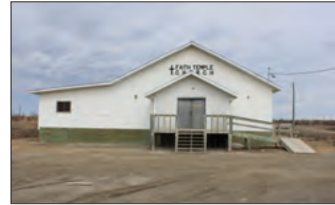
Fig. a94 - Community Church with accessible ramp
