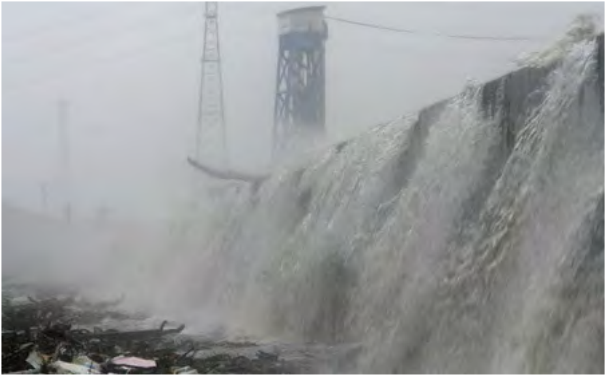
fig. 40: Levee Overtopping at the Industrial Canal
