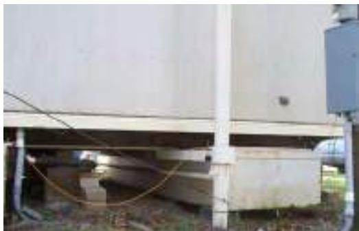
fig. 124: Detail of Amphibious Foundation
