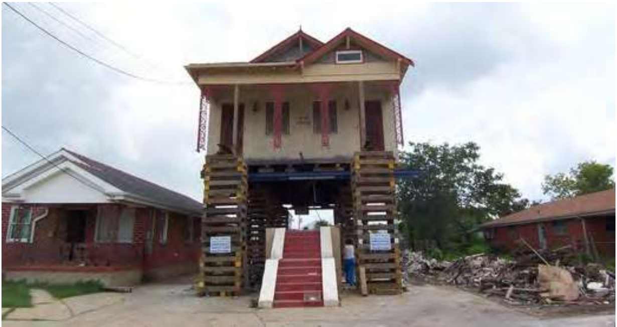
fig. 84: An Elevated Double Shotgun House
