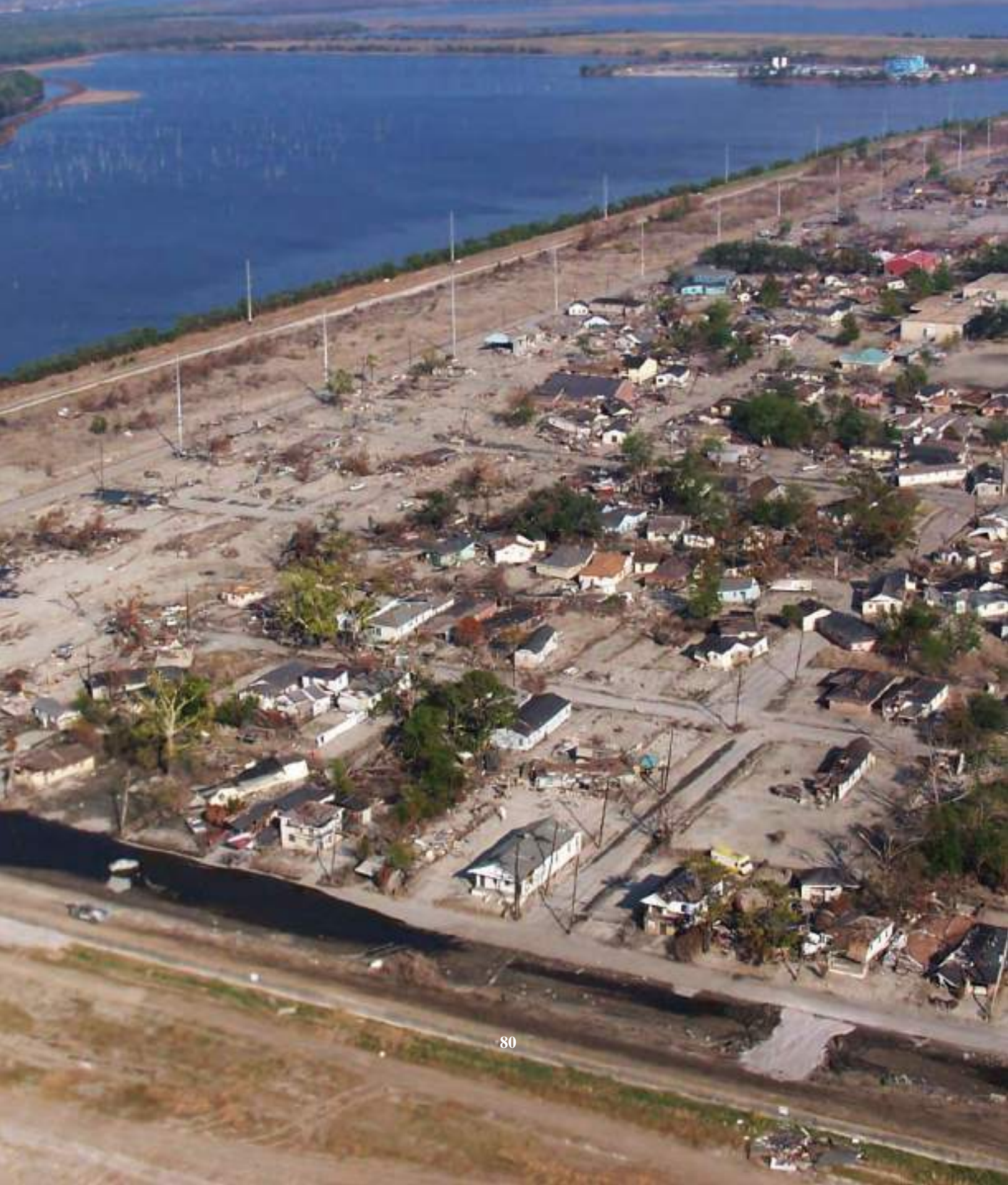
fig. 57: Northern Portion of the Lower Ninth Ward - Post-Katrina New Orleans, 2006
