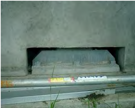
fig. 192: FLOAT House, Base of Vertical Guidance Post, August 2009
