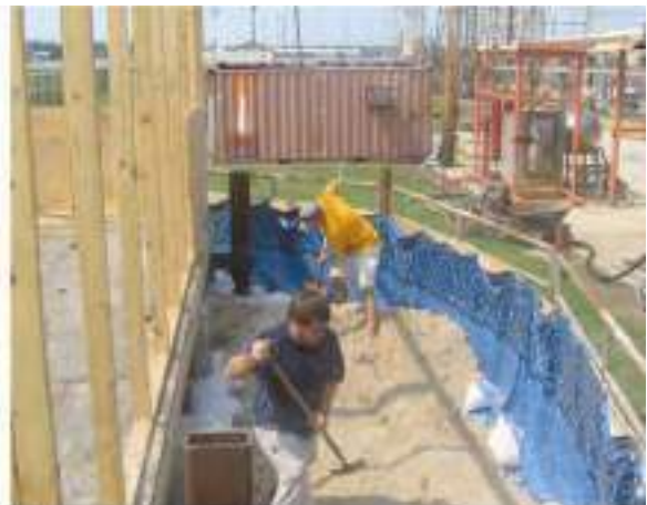
A layer of sand holds down the tank liner
