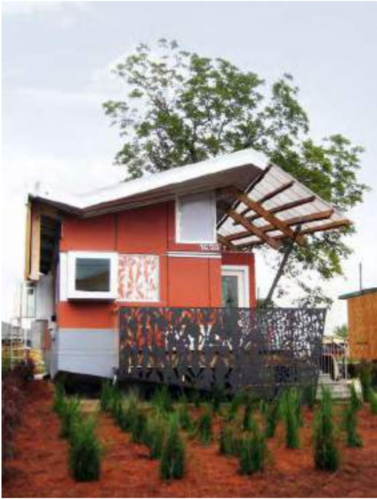
fig. 194: FLOAT House Completed October 6th 2009, Front View
