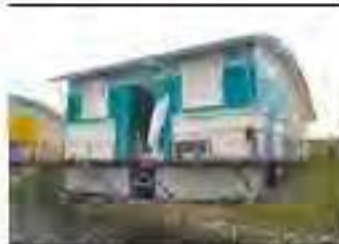
This house in a flood-prone community in the Netherlands has a buoyant foundation to reduce flood damage. The system works like a floating dock. When flooding occurs, the house is lifted above the water by flotation blocks beneath the home. / NNS
