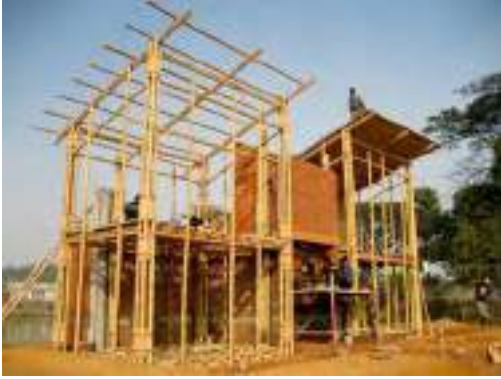
Day 55 – Bamboo frames are erected for both dwellings
