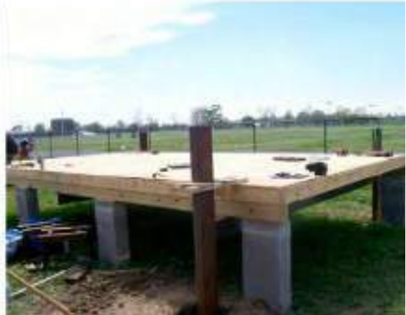
Setting the vertical guidance poles
