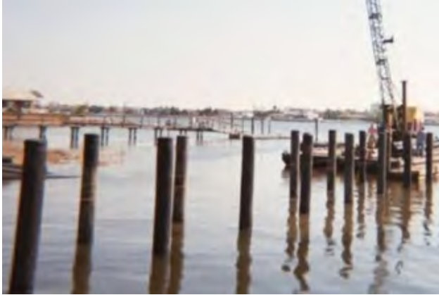
fig. 247: Thermoplastic Timber Piling Installation
