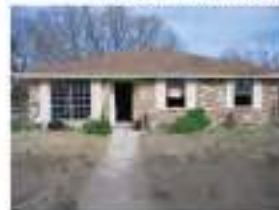
house on slab foundation
