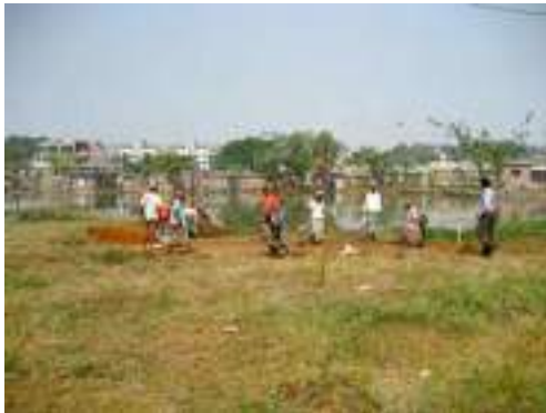
Day 1 – Start of excavation, November 12, 2009
