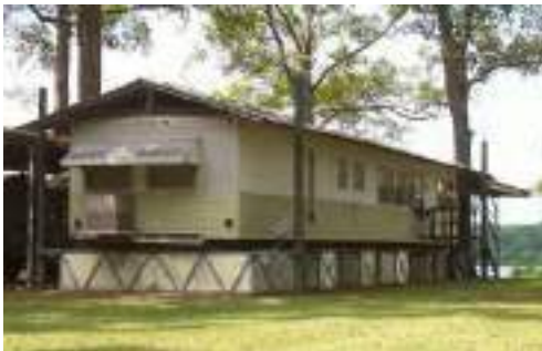
Figure 2: Amphibious houses in rural Louisiana, dry in September, floating in February.
