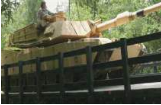
fig. 235: Bridge made of Thermoplastic Timber
