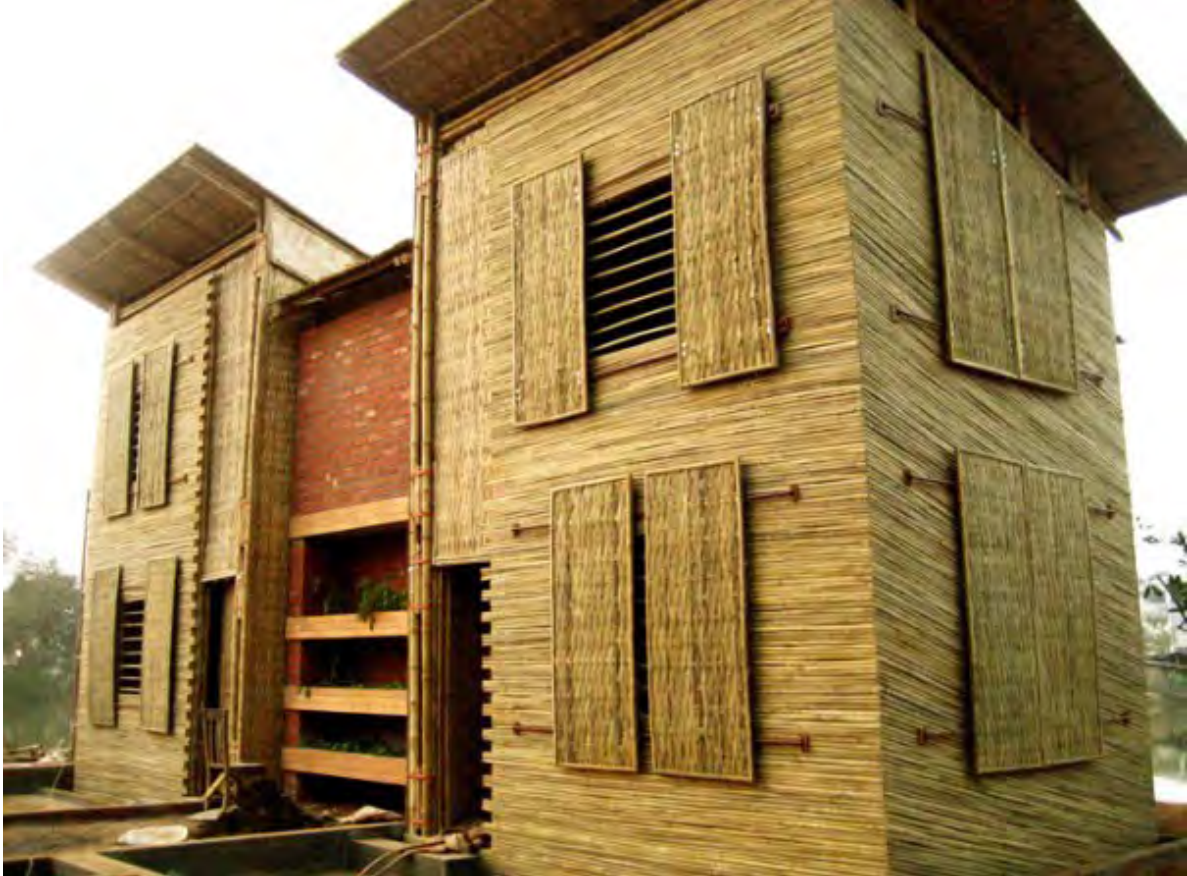
fig. 223: LIFT House, Completed January 2010, Three-Quarter View
