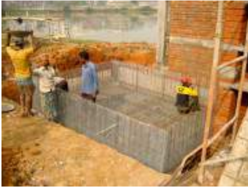
Day 33 – Ferrocement frame prepared for one of the buoyant foundations
