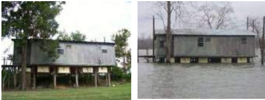
Figure 3: An amphibious house in rural Louisiana, the same house in September and in February.
