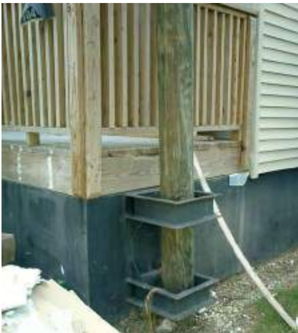
fig. 171: Vertical Guidance Post - Detail
