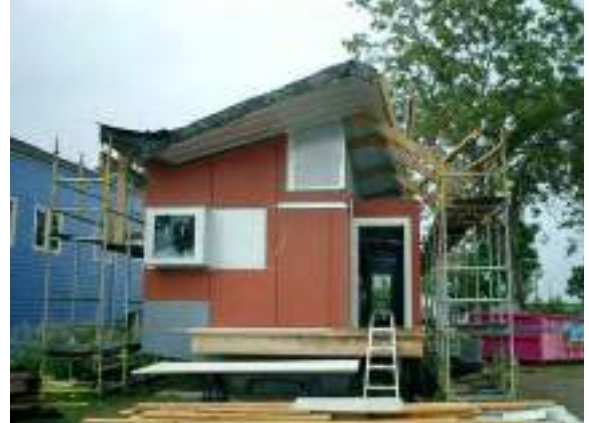
fig. 189: FLOAT House, East View, August 2009
