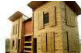
fig. 229: LIFT House, Dhaka, Bangladesh
