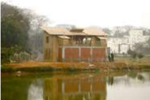
Day 69 – The lift house from across the pond
