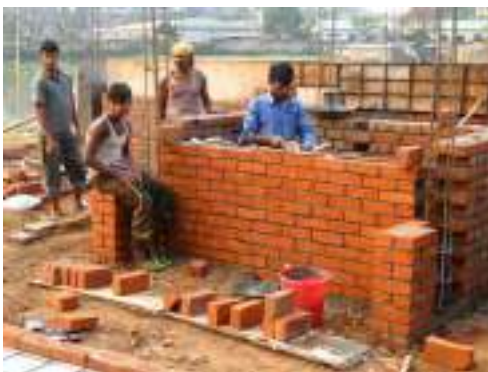
Building up the water storage cistern walls
