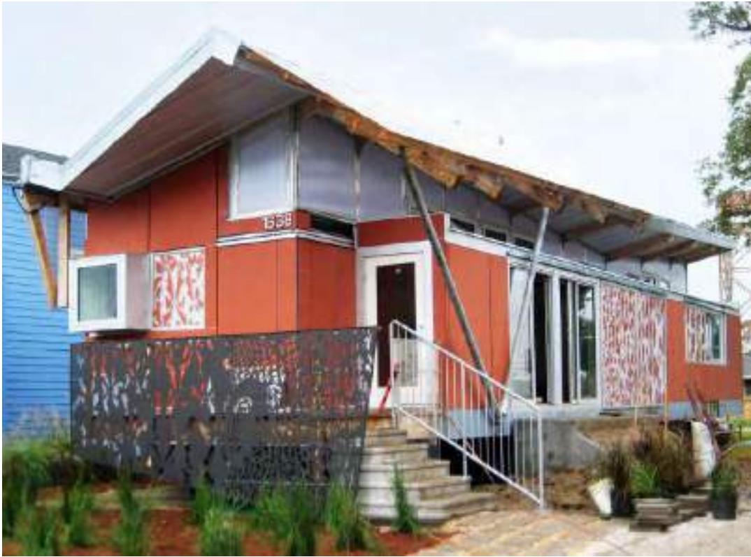
fig. 198: FLOAT House Completed October 6th 2009, Corner View
