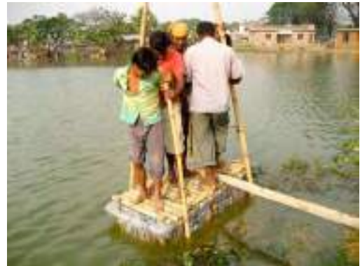
Day 11 – Sample buoyant foundation is tested with live load
