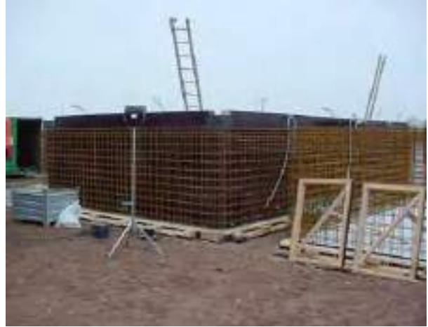
concrete walls of each box are reinforced with steel
