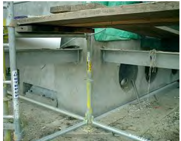
fig. 193: FLOAT House, Foundation, August 2009
