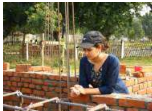
Prithula Prosun supervising construction
