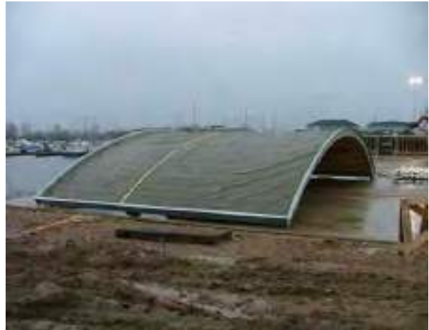
the prefabricated roof is assembled on site
