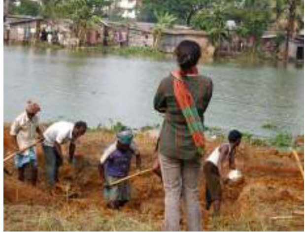
fig. 211: Prithula Overseeing Excavation
