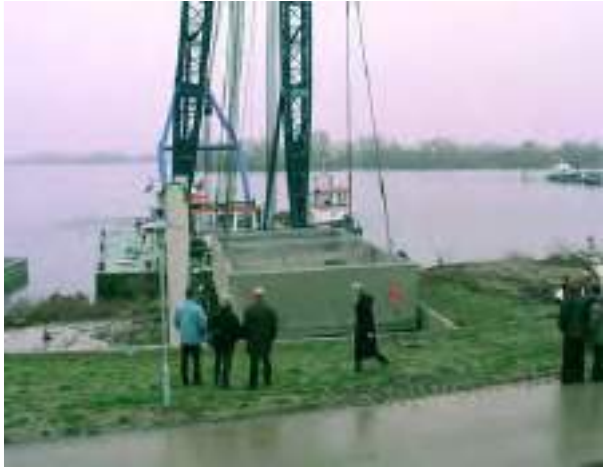
the box is hoisted into its place
