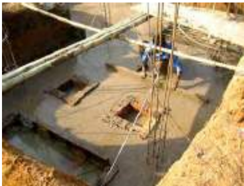
Concrete foundation for the service core
