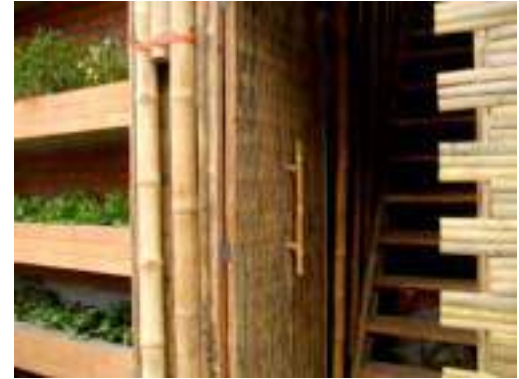
Day 68 – Photo of bamboo entrance door and brick vertical garden
