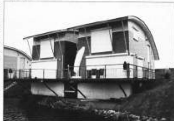
The house in a flood-prone community in the Netherlands has a buoyant foundation to reduce flood damage. The system works like a floating dock.
