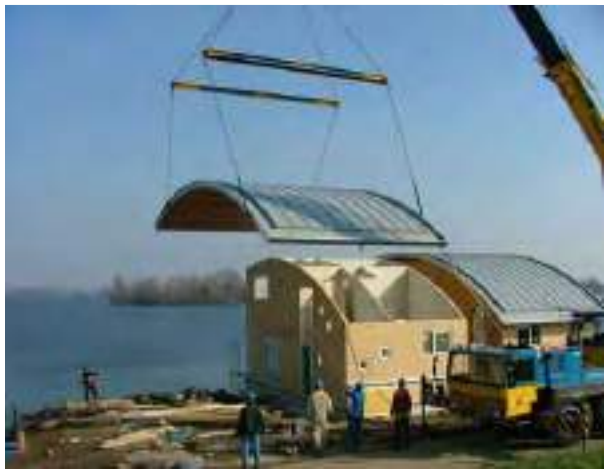
the roof is hoisted on top of the prefabricated wooden-frame houses
