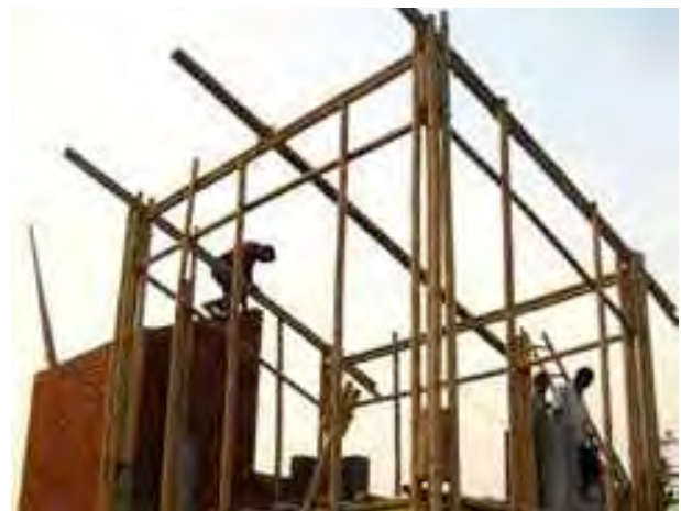
fig. 219: Bamboo Structure in Place
