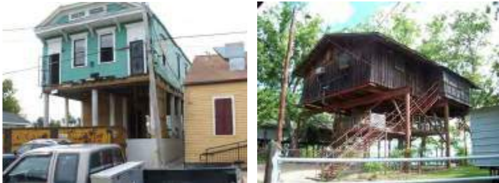
Figure 1: Permanent static elevation of homes in south Louisiana. This is the flood mitigation strategy currently promoted by US government agencies.
