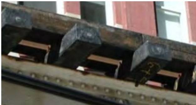
fig. 248: Elevated Rail in Chicago Using Thermoplastic Ties
