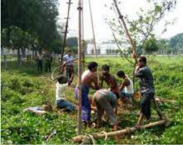
fig. 210: Digging Bore Hole for Soil Test
