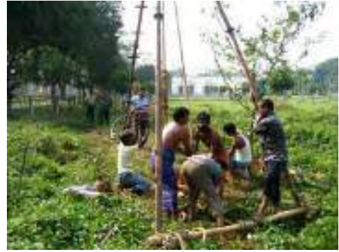
DHAKA: November 2009 – Soils testing before the start of construction
