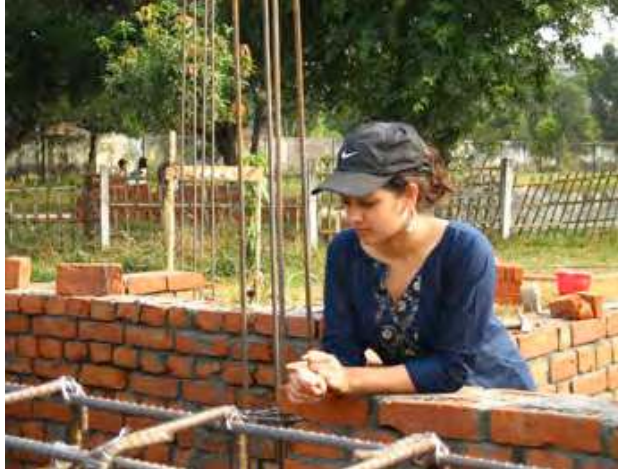
fig. 216: Prithula Overseeing Wall Construction
