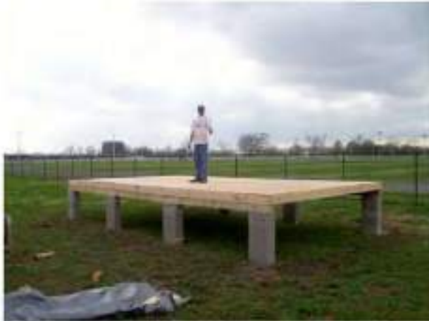
Building the platform
