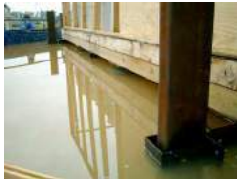
Buoyant foundation at rest on the water
