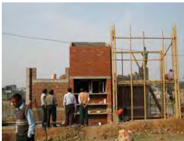
fig. 220: Bamboo Structure in Place beside Concrete Spine
