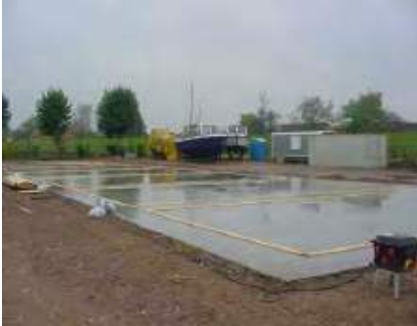
concrete box is measured out on the concrete workspace on site
