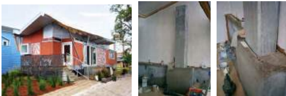
Figure 4: The FLOAT House, New Orleans. Elevation, interior guide post and sleeve detail.
