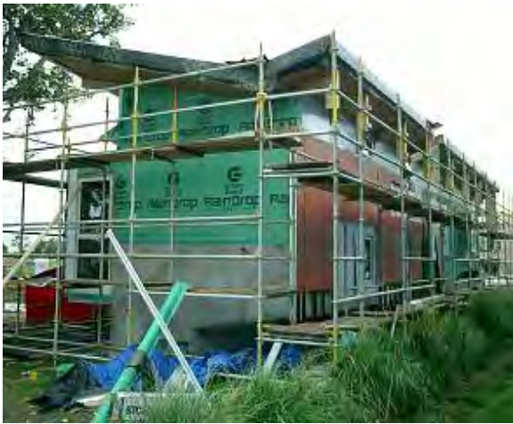
fig. 190: FLOAT House, Scaffolding on South West Perspective, August 2009
