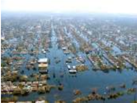
New Orleans after Hurricane Katrina
