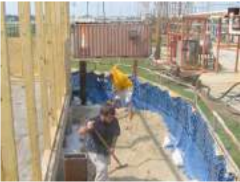
A layer of sand holds down the liner
