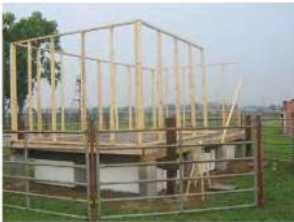
Adding the house frame and flood tank
