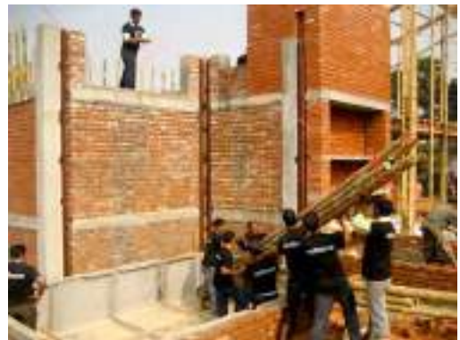
Day 50 – Pre-fabricated bamboo columns for second dwelling are erected
