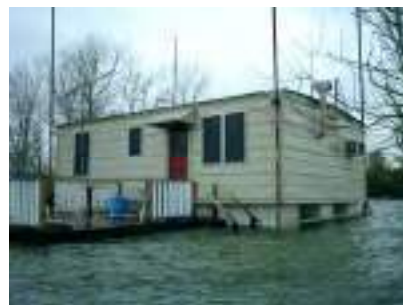
Figure 2: Amphibious houses in rural Louisiana, dry in September, floating in February.
