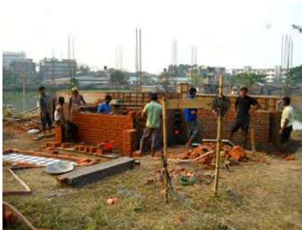
fig. 218: Construction Team Assembling Masonry Wall
