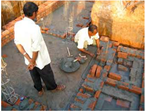
fig. 213: Preparing Foundation
