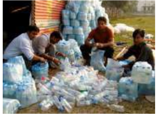
Day 40 – Empty used water bottles are prepared for second buoyant foundation
