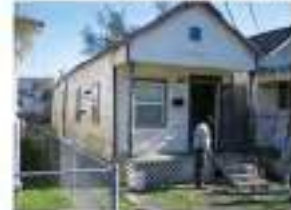
house on pier foundation
