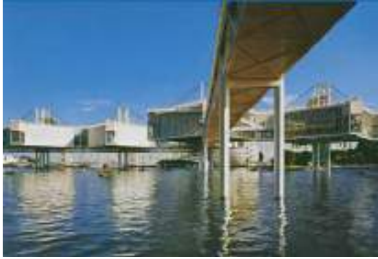
fig. 283: Ontario Place Elevated Walk, Canada
