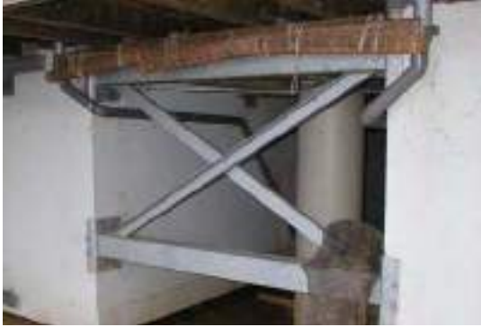
fig. 140: Vertical Guidance Post Connection
