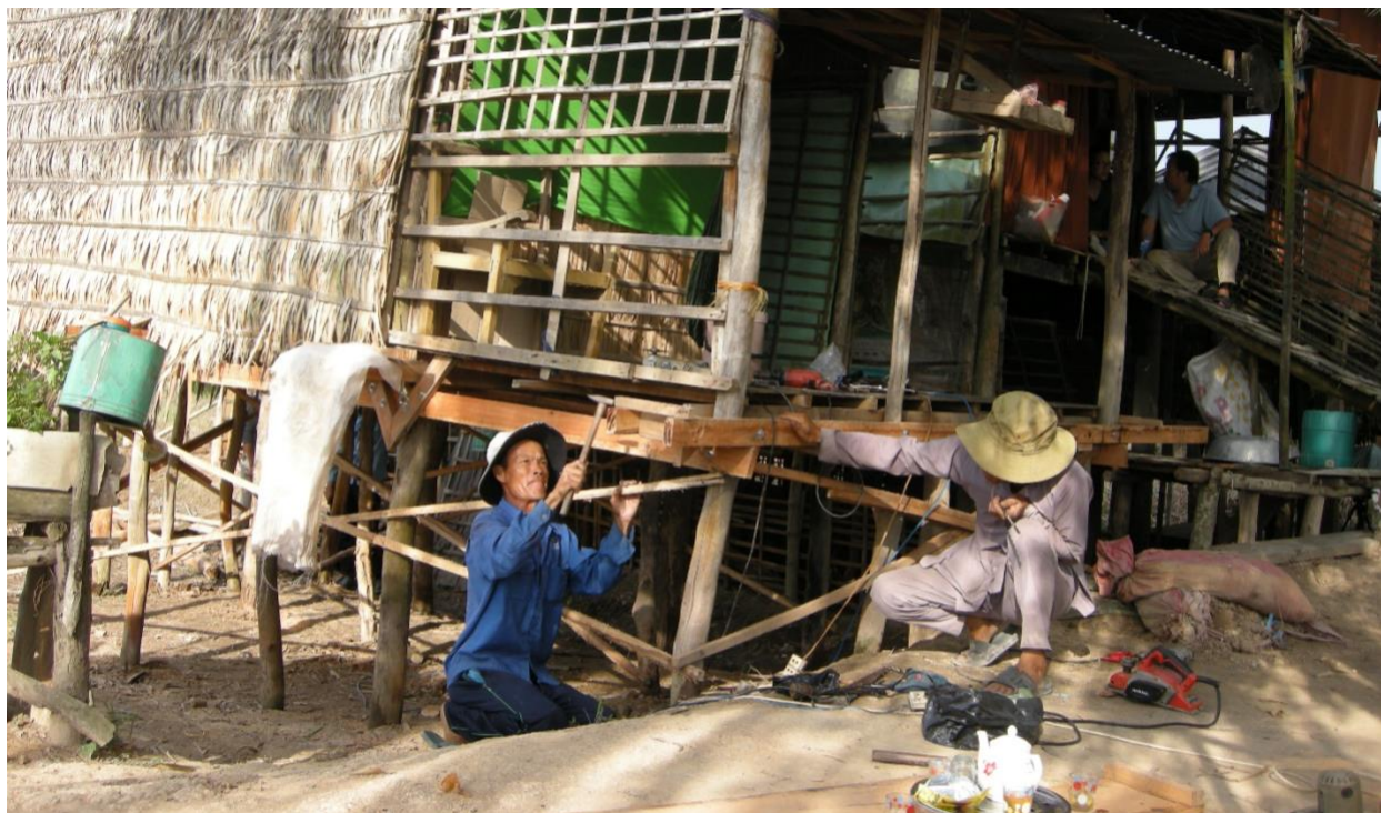
Figure 4 Carpenters retrofitting Nguyen Thi Dung's home in Long An Province.
