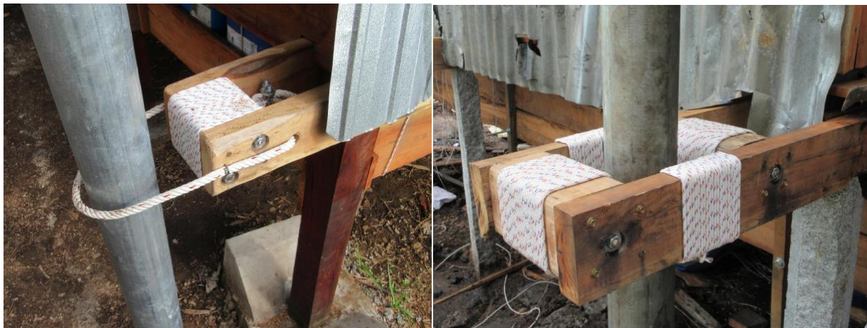
Figure 14 Different methods of construction for sleeves around the vertical guidance posts. On the left is a rope sleeve that loops around a vertical guidance post on Nao's house and on the right is a wood box sleeve with rope cushioning on Lac's house.
