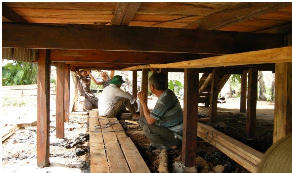
Figure 24 Retrofitting underneath Dang Van Nang's house in Long An.
