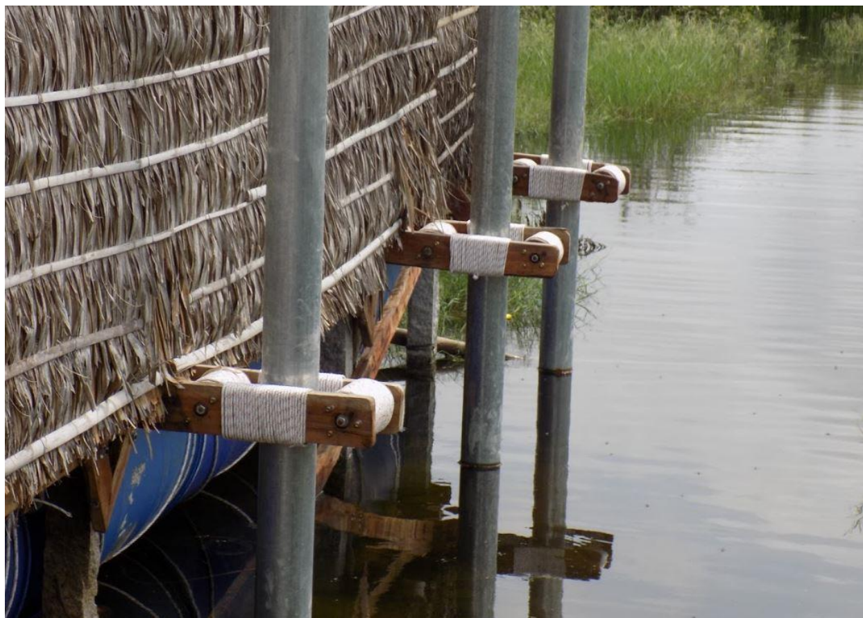
Figure 19 Centering devices and vertical guidance posts along Nguyen Van Lac's home in An Giang.
