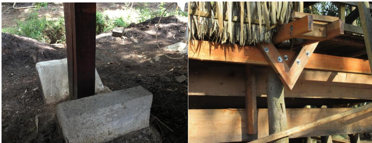
Figure 15 Different methods of construction for centering devices. Nguyen Van Nao's house is on the left and Nguyen Thi Dung's house on the right.
