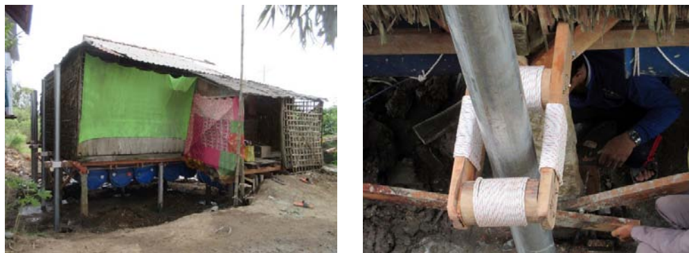
Figure 7: Dang Van Nang's house (left) and the more complex sleeve detail (right) (BFP / Elizabeth English)
