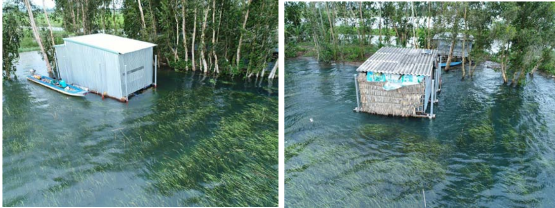
Figure 8: Amphibiated homes in An Giang Province floating on the 2018 monsoon flood (Pham Duy Tien)
