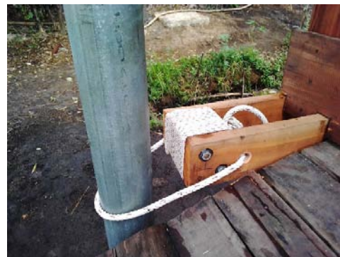
Figure 5: Nguyen Van Nao's house, a new built house (left) and the sleeve detail used (right) (BFP / Elizabeth English)
