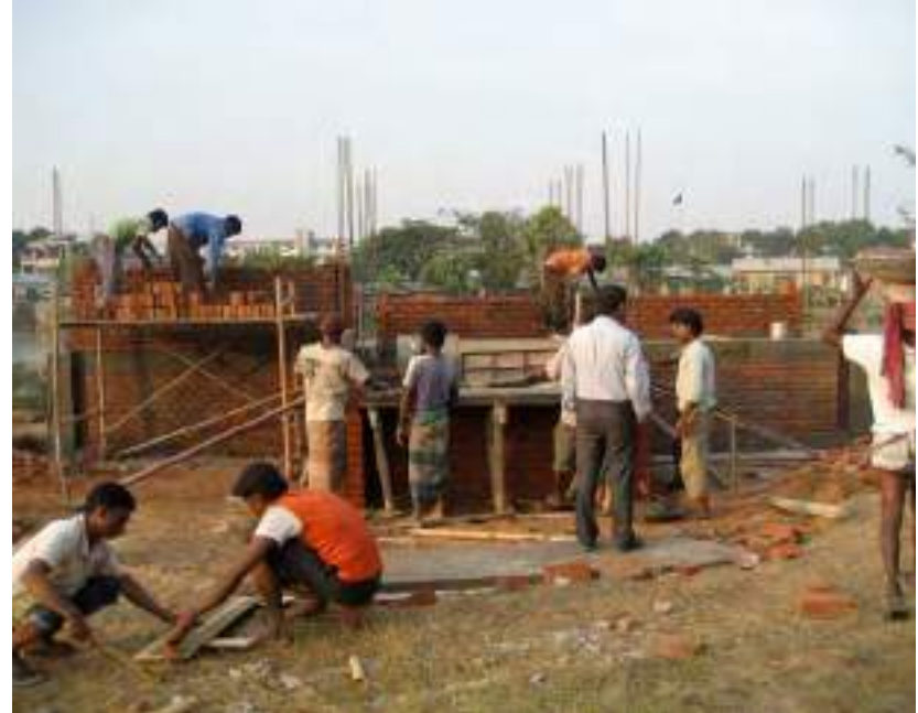
8.54. Workers laying brick walls above the lintel band
