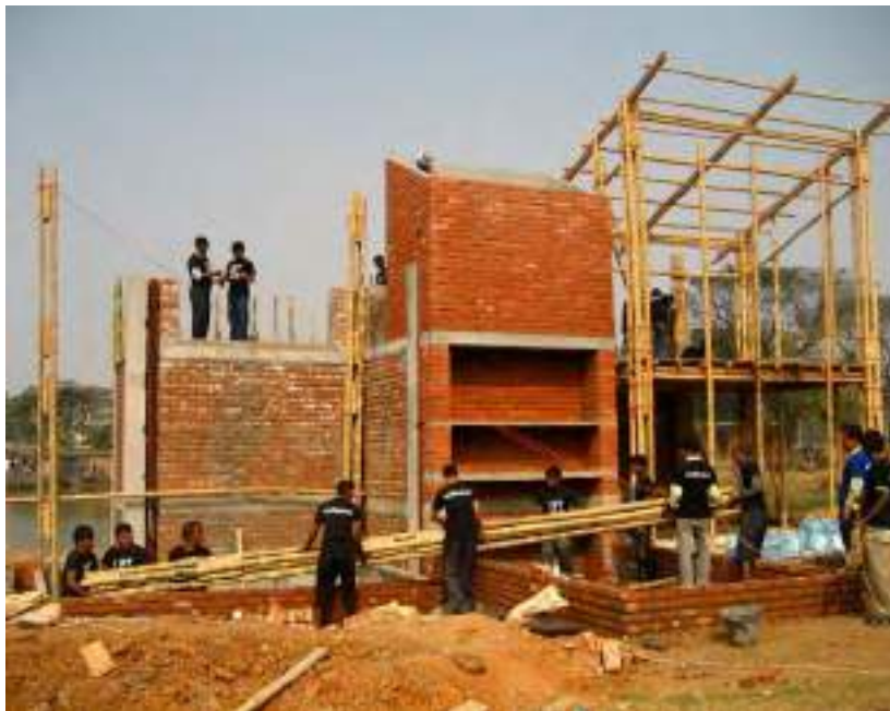
8.105. Second bamboo frame under construction
