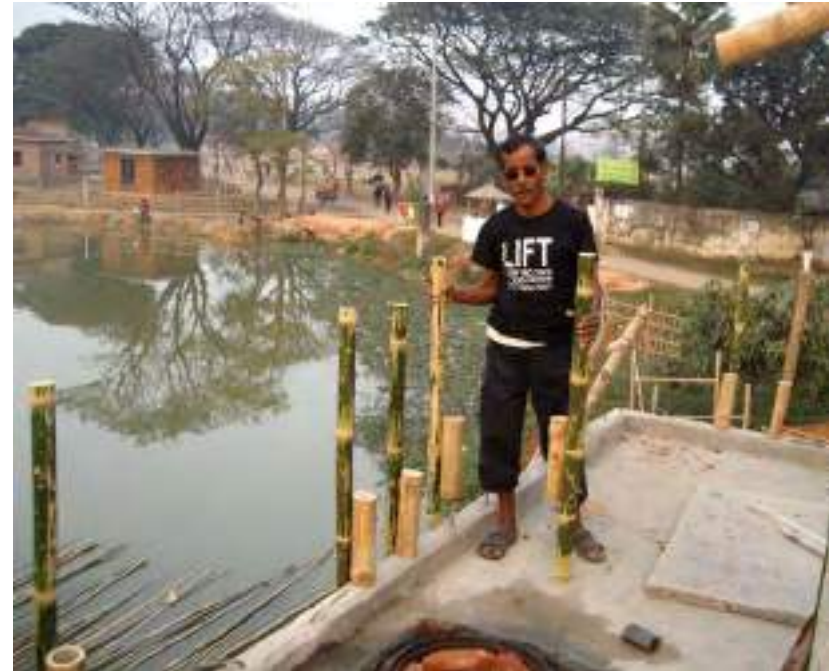
8.98. Installment of bamboo railings
