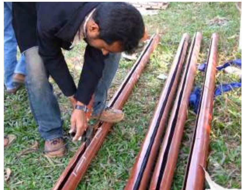
8.76. Straightening the opening in the steel vertical guidance tracks
