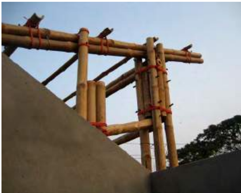
8.101. Bamboo frame showing connections
