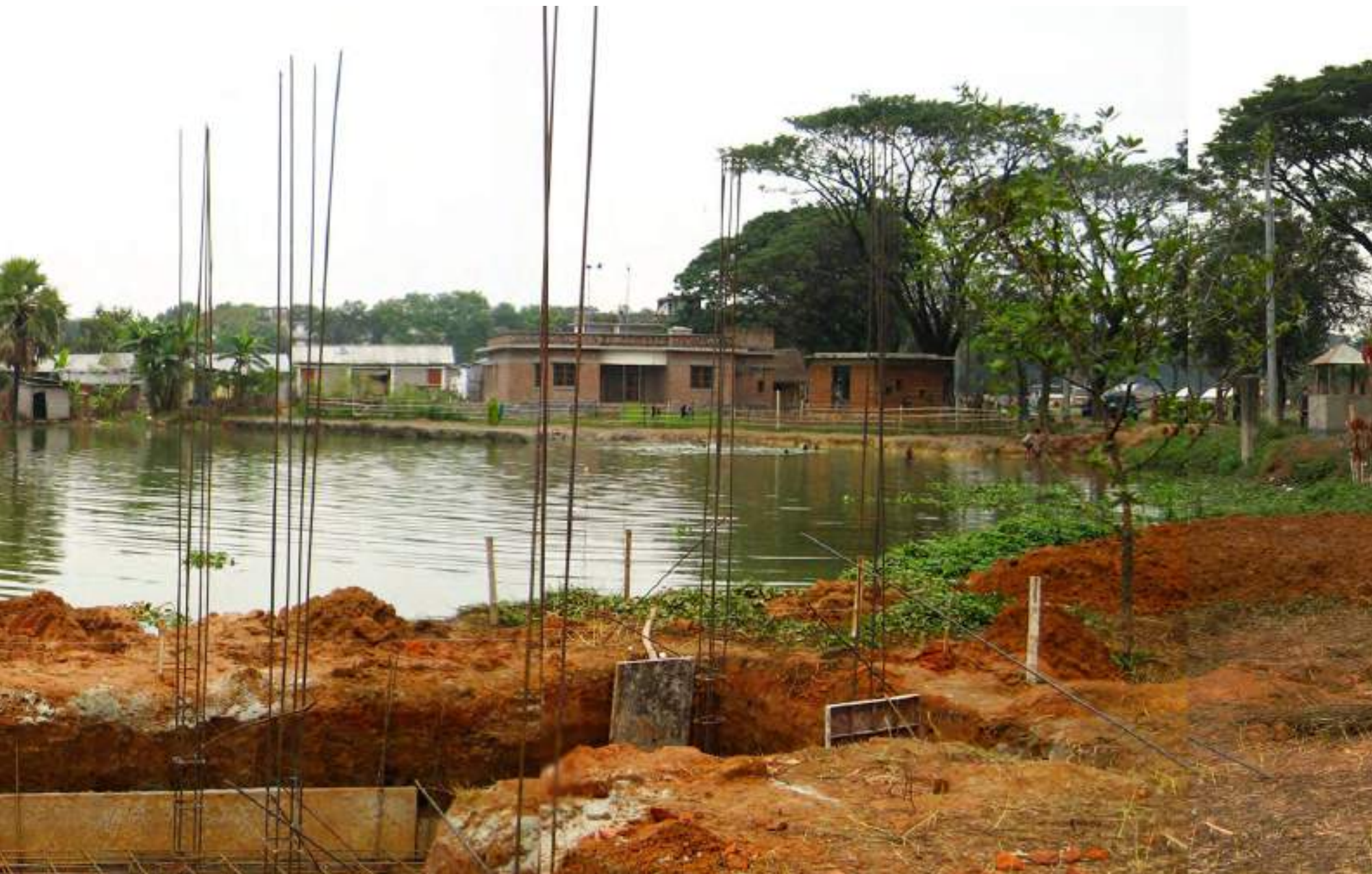
8.26. Panoramic photo of LIFT site with reinforcement bars for columns
