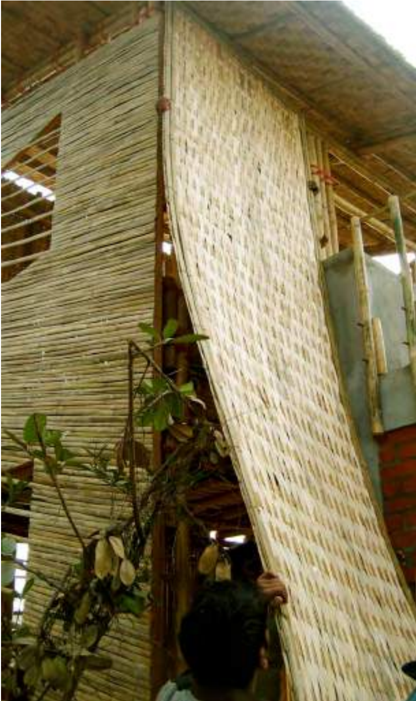
8.135. Installation of interior wall
