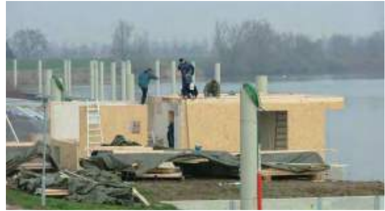
5.7. Ground floor completed of the amphibious houses
