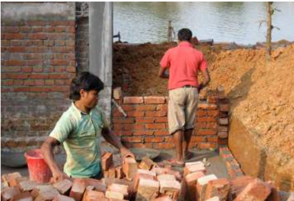
8.58. Side walls for water bottle foundation dwelling holding tank
