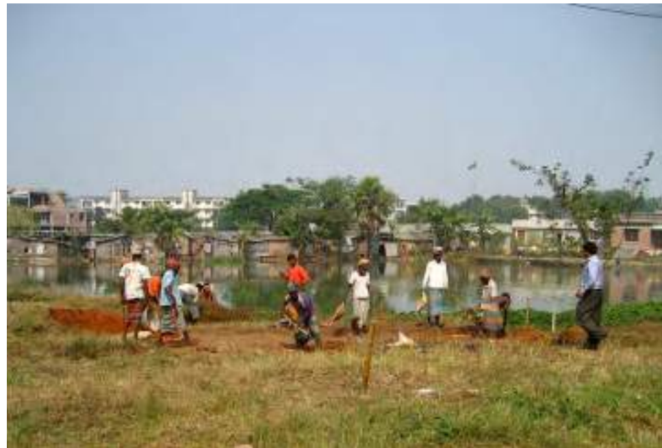
8.1. Excavation for the LIFT house service spine
