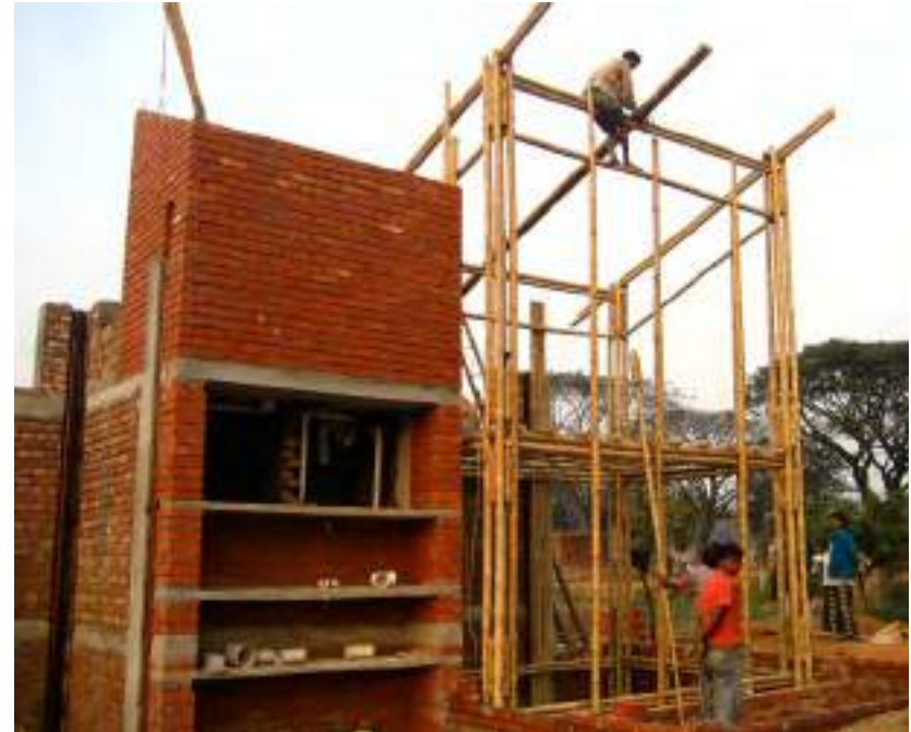
8.88. Service spine finished and installment of first bamboo structure complete
