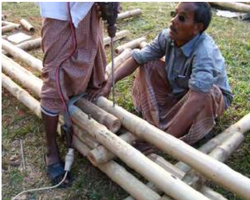
8.74. Bamboo pre-drilled before inserting steel rod into columns
