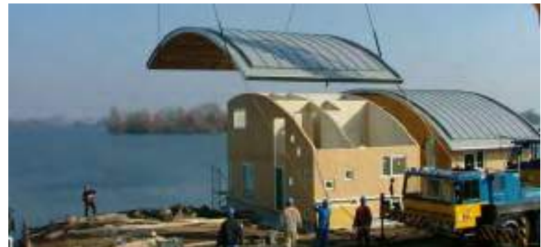
5.9. Roof installation on amphibious houses
