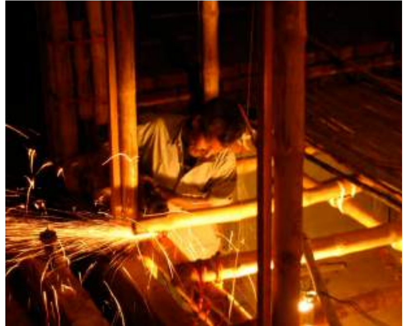
8.120. Installment of floor joists in ferrocement foundation
