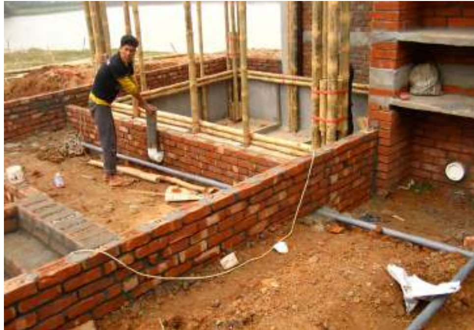
8.115. Plumbing laid for drainage
