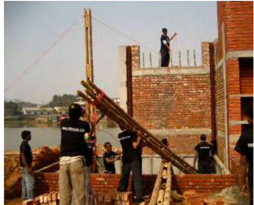
8.102. Columns pulled in place on ferrocement foundation
