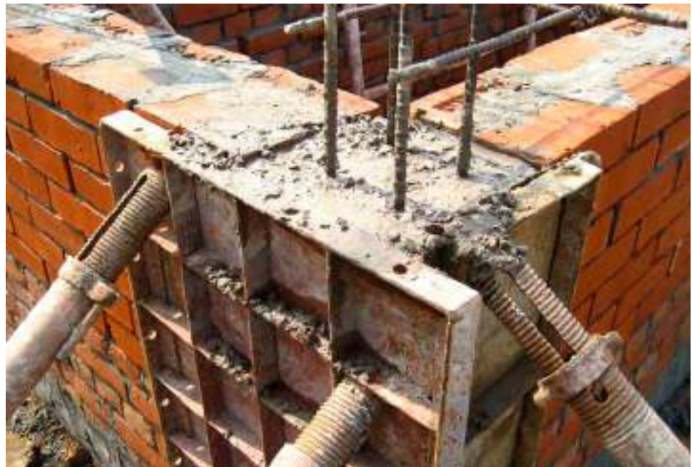
8.50. Shutters around the corner concrete columns in the service spine
