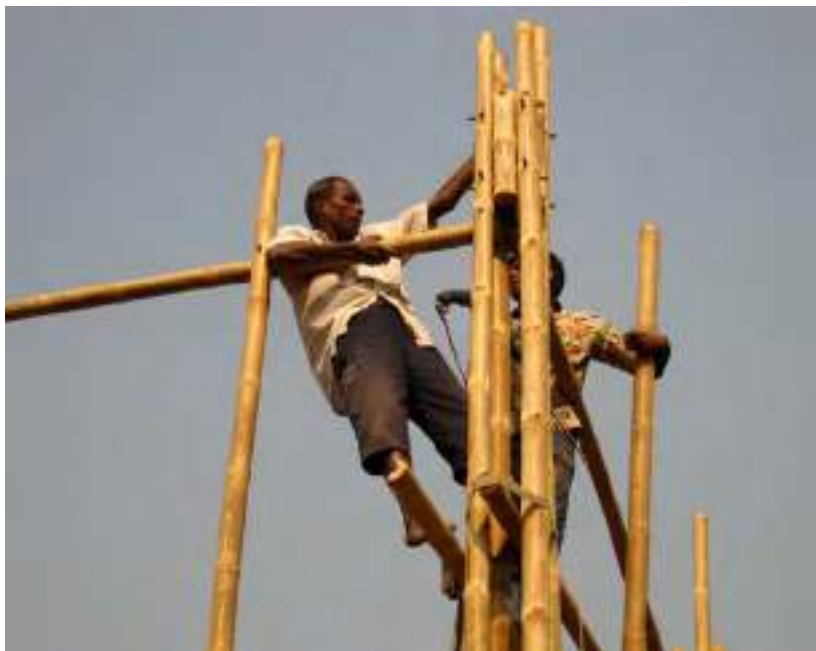
8.80. Beams attached to columns by bamboo workers
