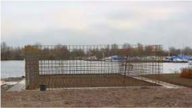
5.4. Reinforcement for the amphibious foundation
