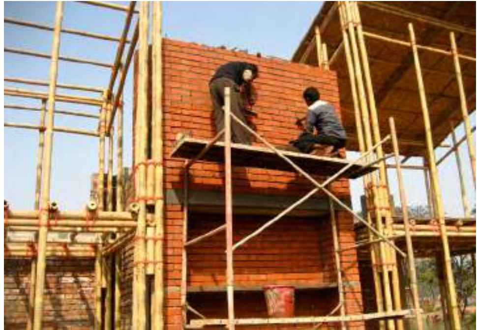
8.108. Grout lines cleaned by workers
