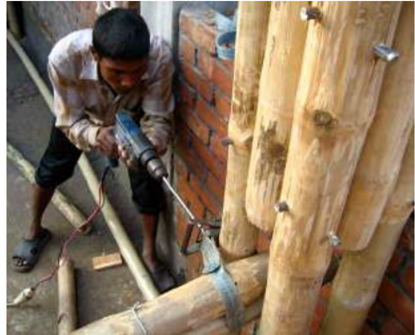
8.81. Connection of bamboo beam and column
