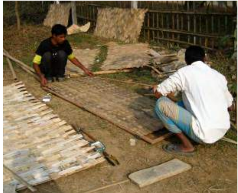
8.142. Sliding window shutters being prepared by bamboo weavers
