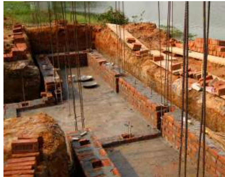
7.1. Perimeter brick wall under construction
