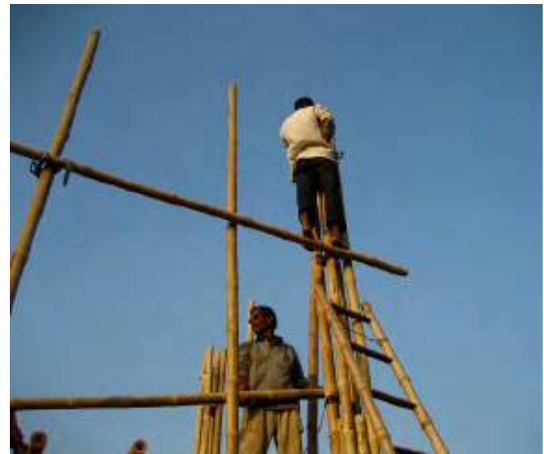
8.85. Installment of top beams
