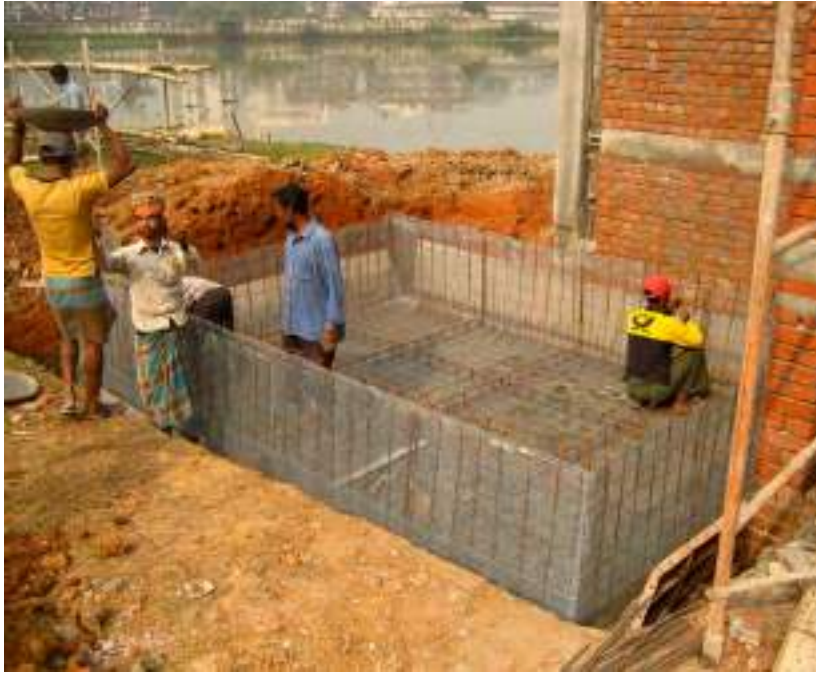
8.61. Ferrocement foundation placed into holding tank
