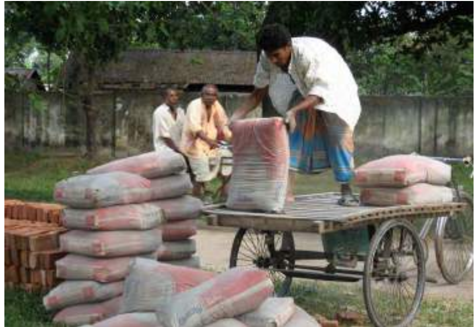
8.22. Cement bags delivered in small amounts to avoid storage on site
