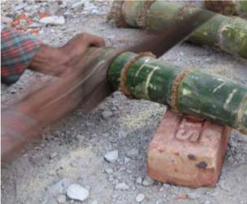
8.45. Bamboo cut by hand saws
