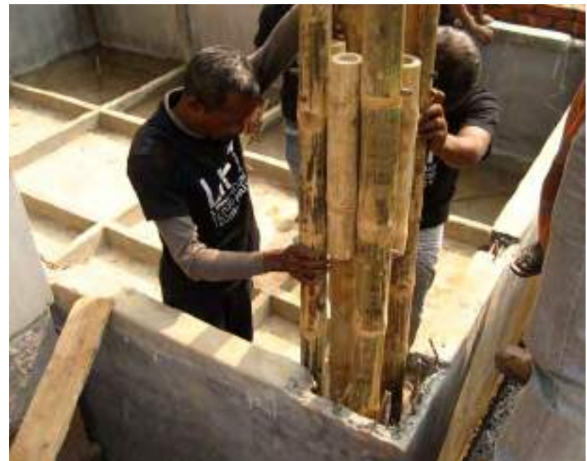
8.99. Careful placement of bamboo column into ferrocement foundation
