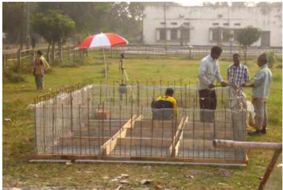
8.60. Ferrocement foundation structural frame
