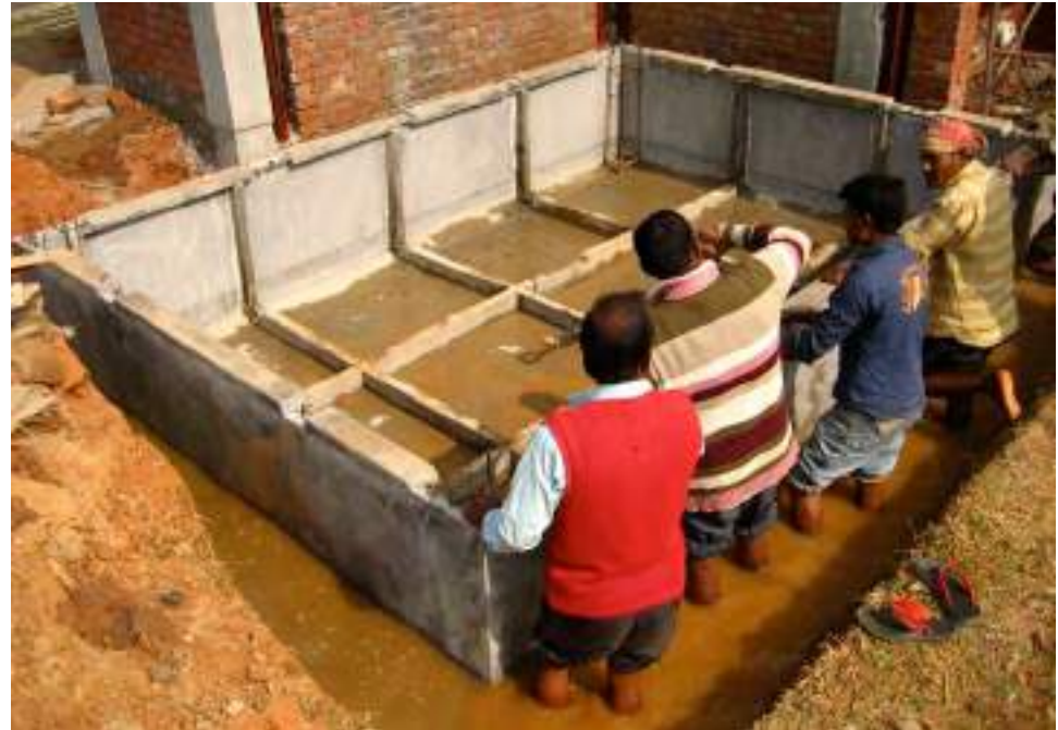
8.94. Ferrocement foundation moved into position after curing
