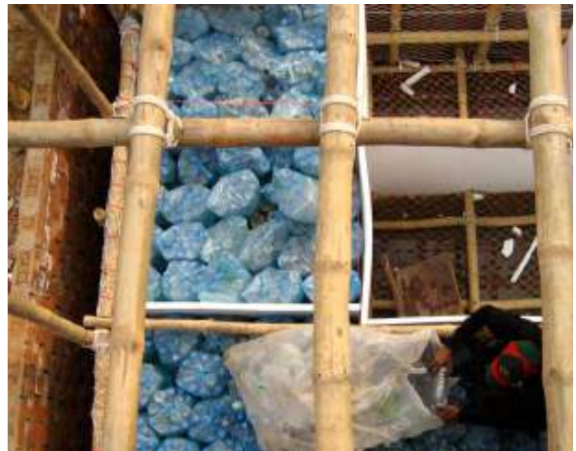
8.107. Used water bottles inserted into foundation
