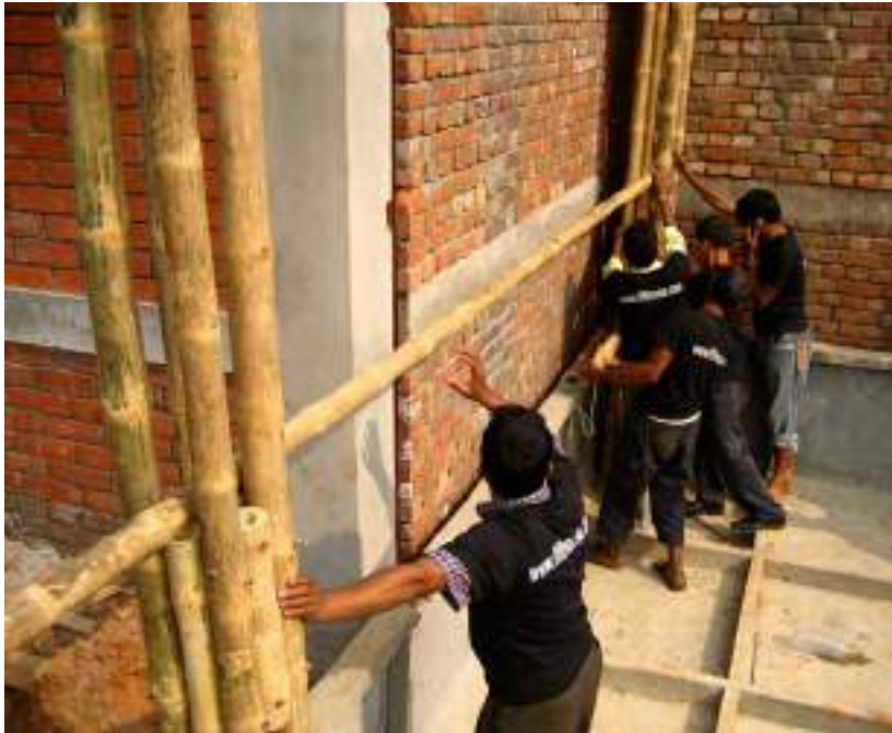
8.100. Beam placement in ferrocement foundation dwelling
