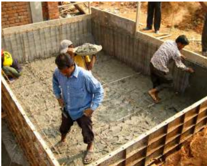
8.62. Cement mixture poured into frame and compressed
