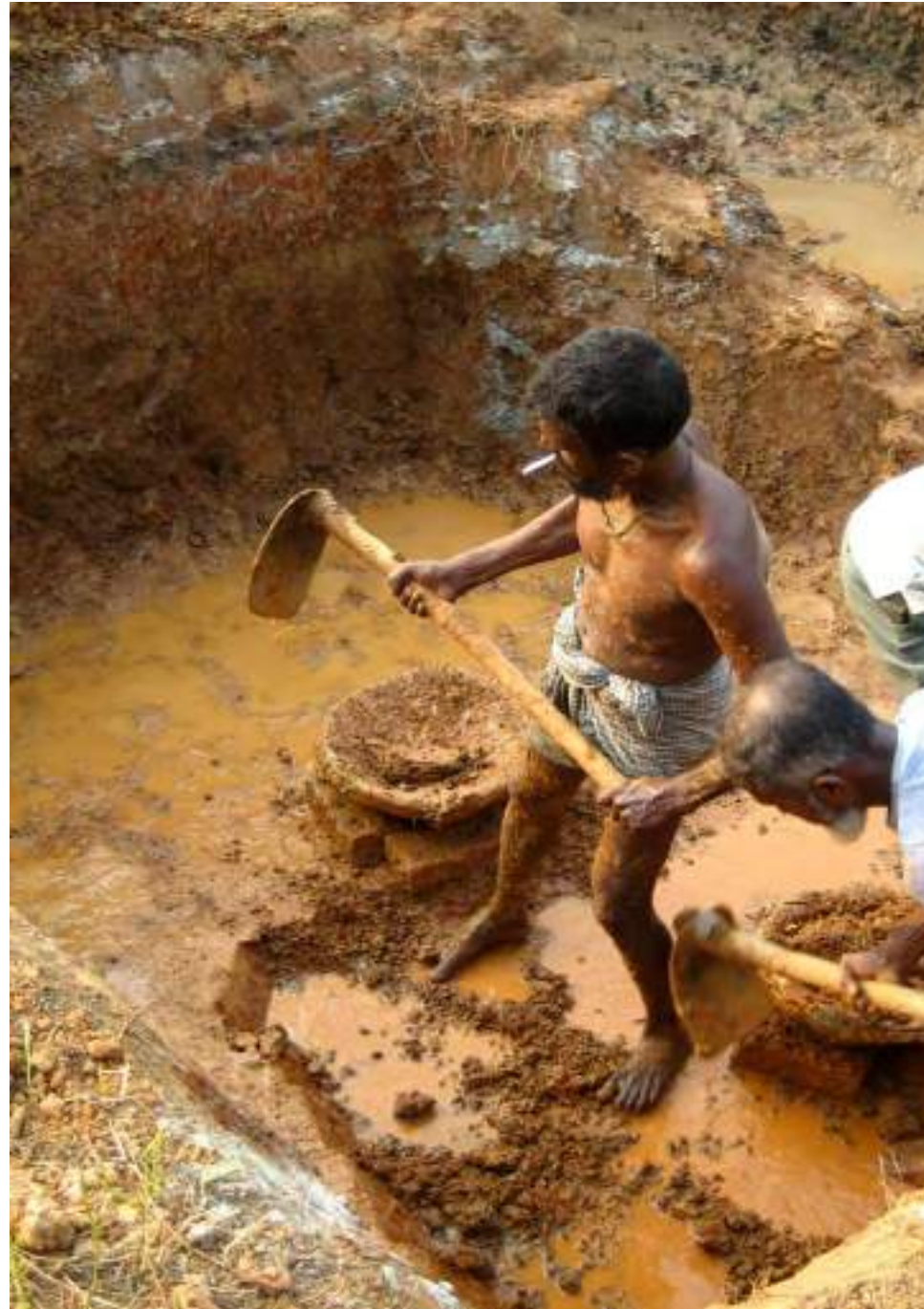
8.19. Excavators faced difficulty in continuing work with the slippery soil
