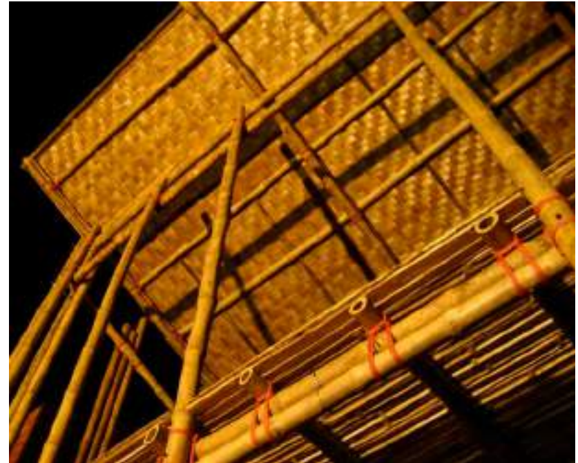
8.113. Bamboo frame with roof
