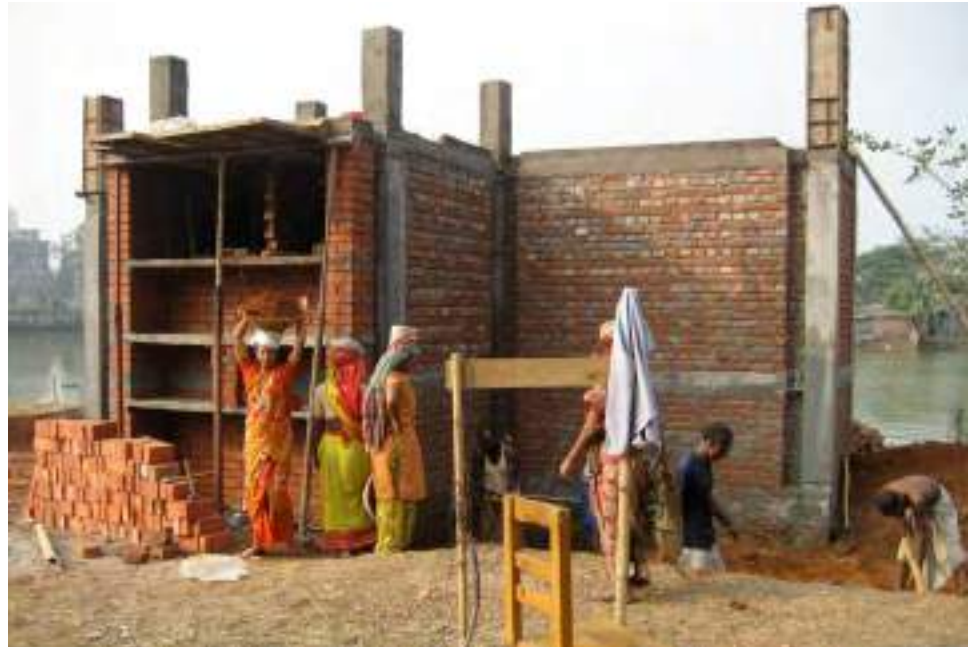
8.56. Excavation of the holding tank for the water bottle foundation dwelling
