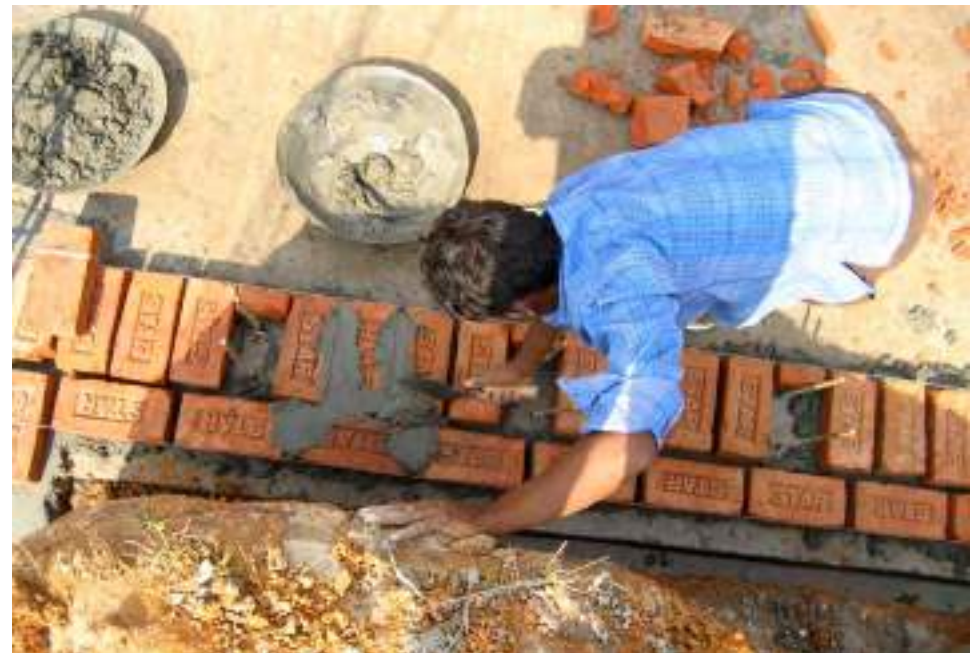
8.28. 15” perimeter wall with dowels for added strength
