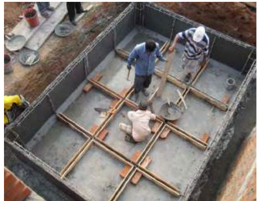
8.64. Shutters laid for concrete ribs
