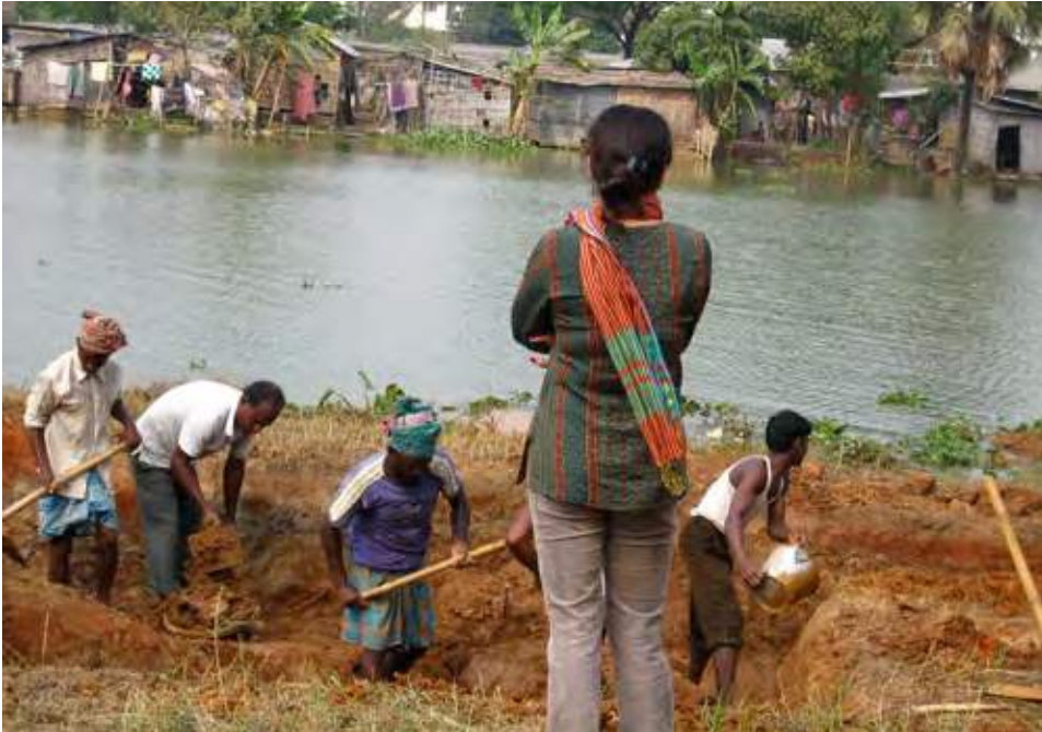
8.14. Beginning of excavation
