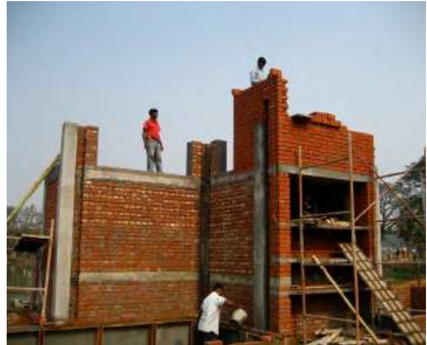
8.75. Grooves left in wall of the service spine to place vertical guidance tracks
