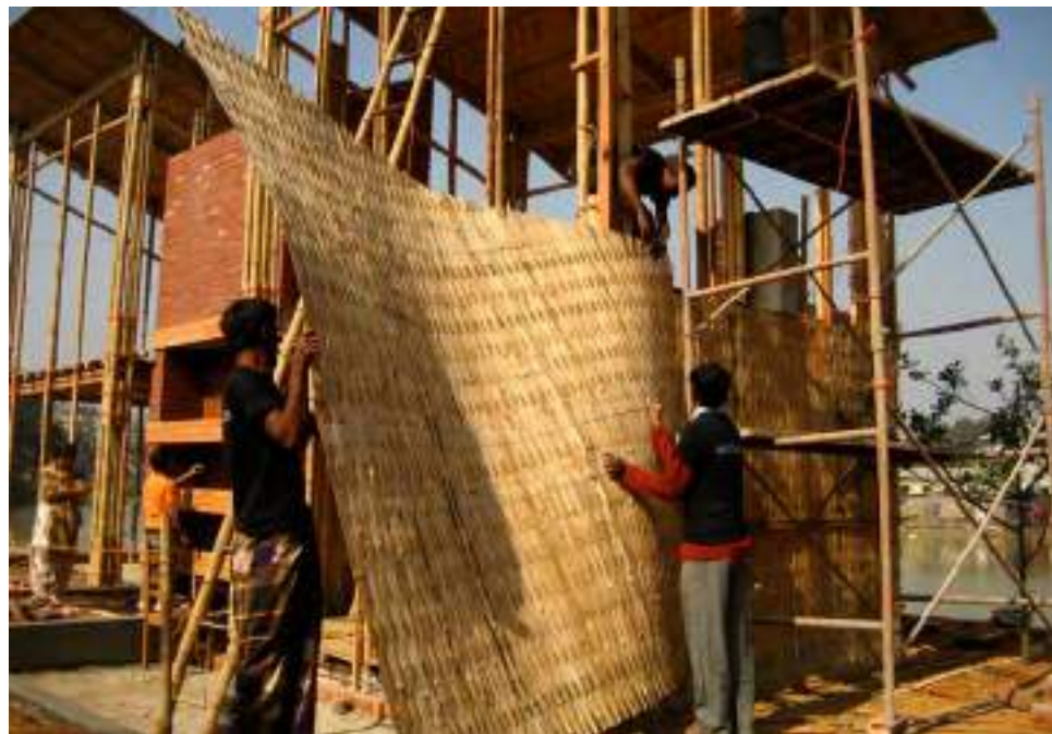
8.116. Installation of interior bamboo wall
