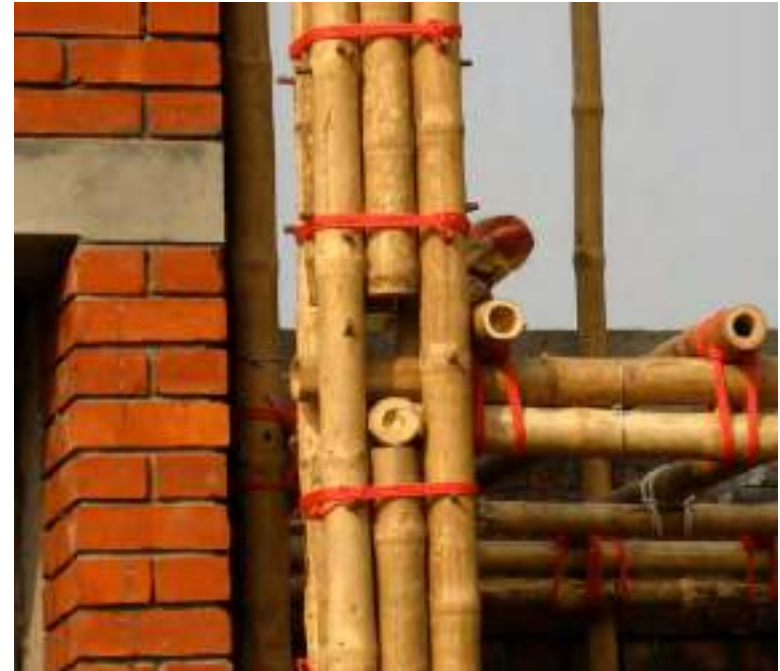
8.84. Detail of column and beam connection
