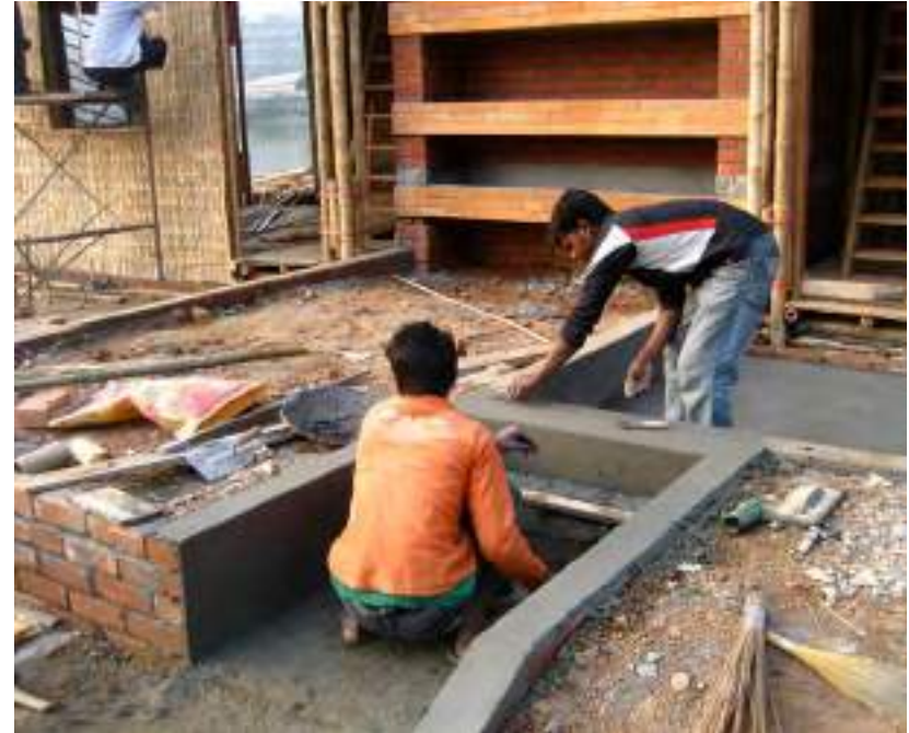
8.131. Construction of front steps
