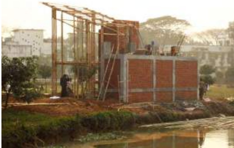
8.104. View of LIFT house across the pond
