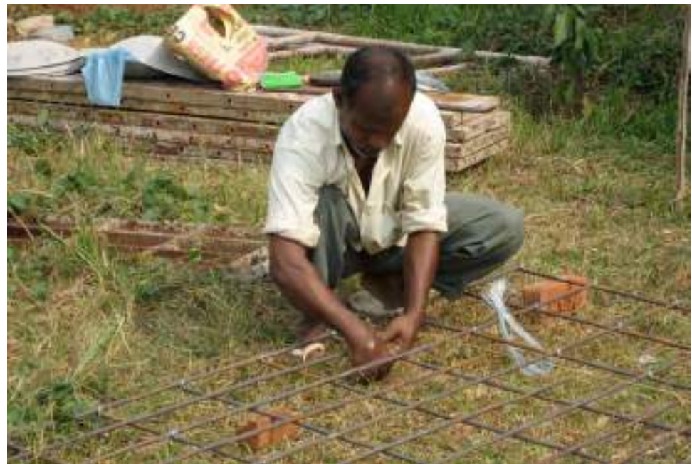
8.23. Reinforcing bars prepared for concrete slab
