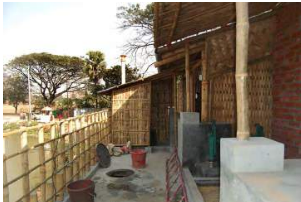
8.139. Shared exterior space on top of service spine
