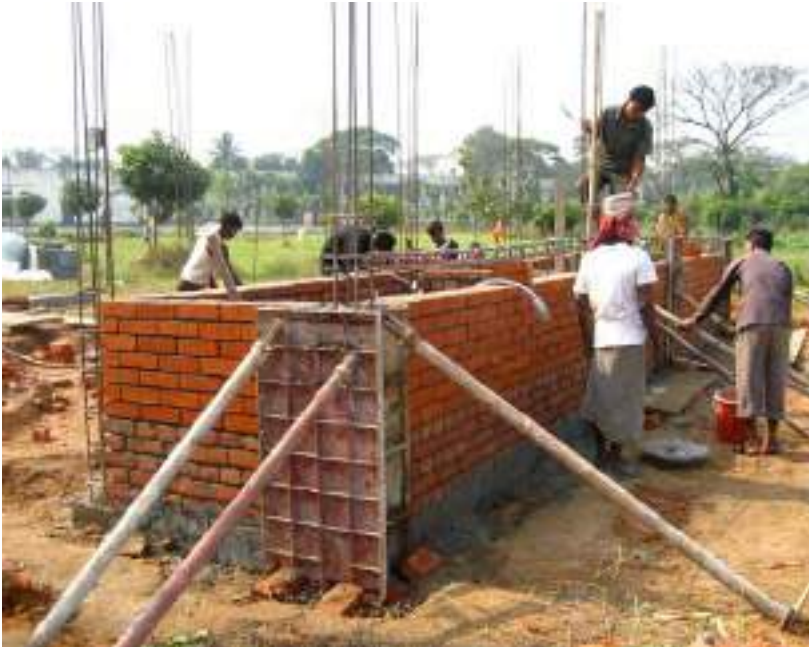
8.52. Ceramic bricks installed in the visible sections above the "Bangla" bricks
