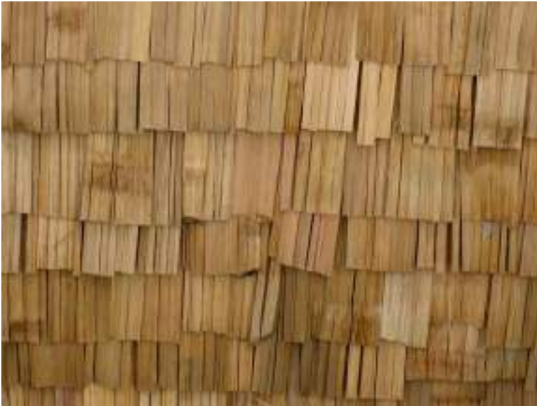
7.15. Sample top layer of bamboo roof
