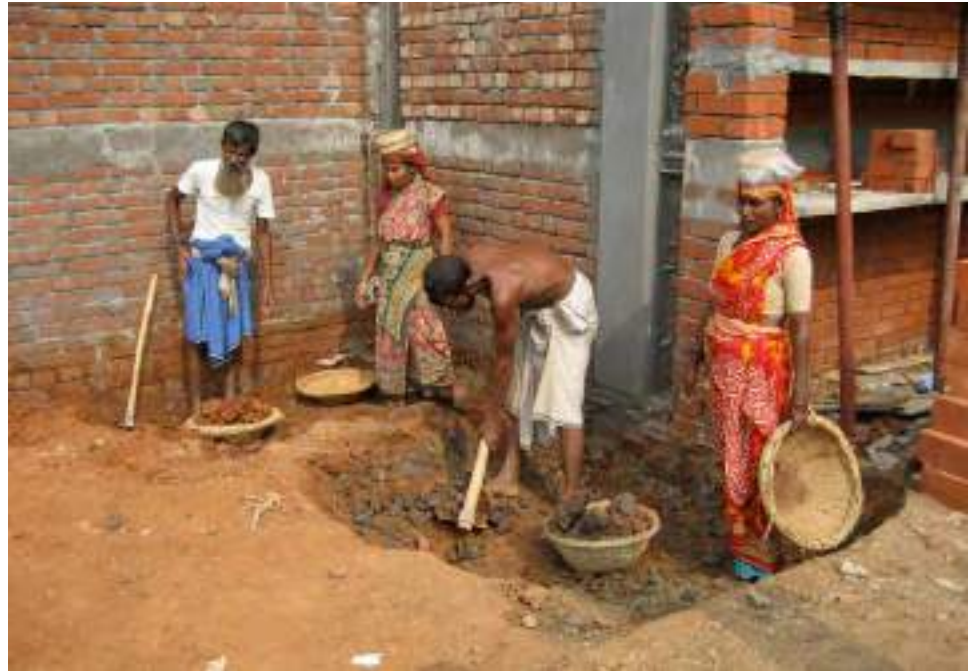
8.55. Excavation of the holding tank for the ferrocement foundation dwelling
