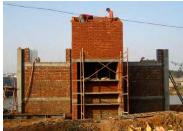
7.2. Service spine under construction with two horizontal lintel bands
