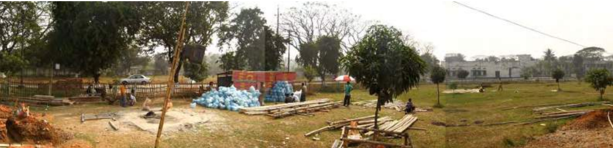
8.93. Panoramic photo of the LIFT construction site
