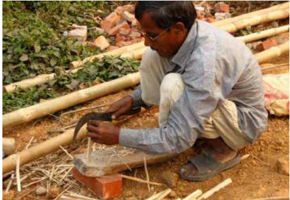
8.77. Bamboo pegs made for joints that will be exposed to water
