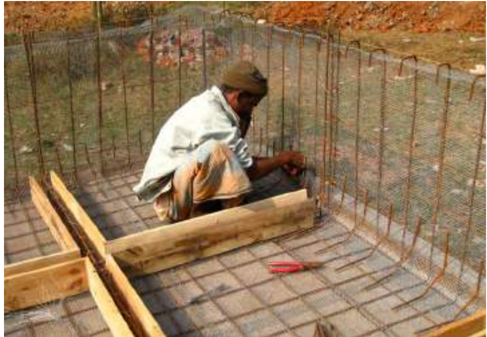
8.59. Ferrocement foundation frame of steel rods and wire mesh
