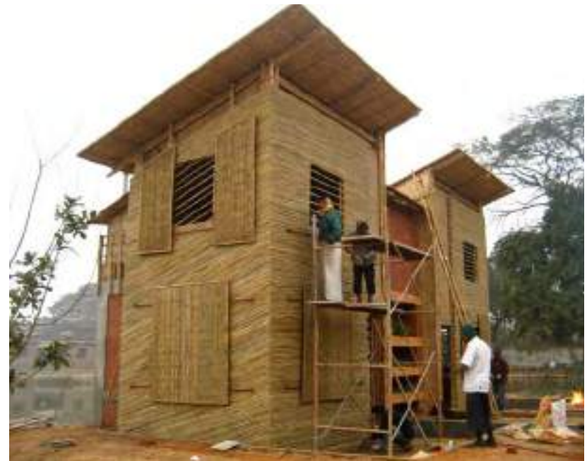
8.148. Installation of sliding shutters
