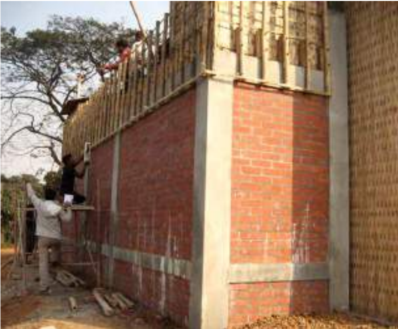
8.140. Railings being secured
