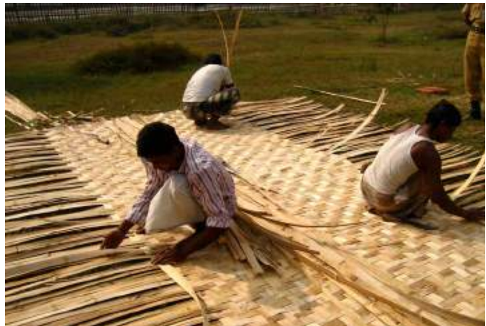
8.95. Bamboo mats woven for interior walls
