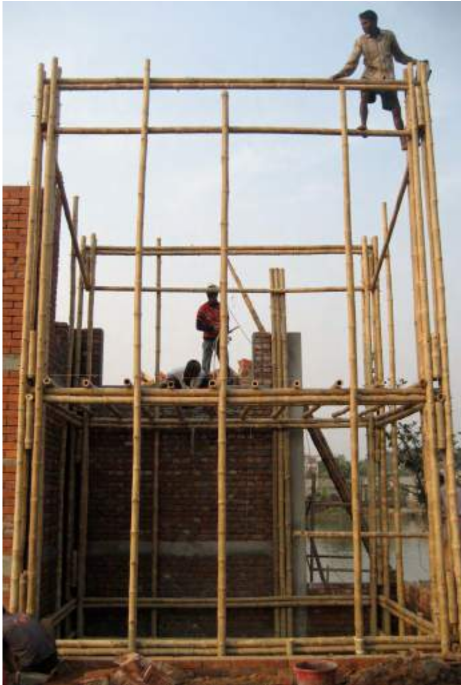
8.83. Structural frame for water bottle foundation dwelling
