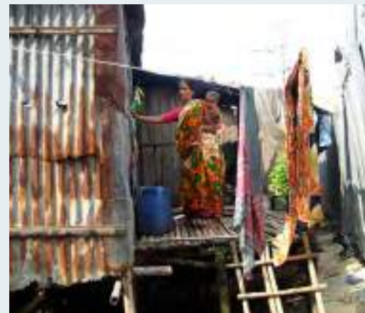
7.18. A corrugated tin house in Karail baste
