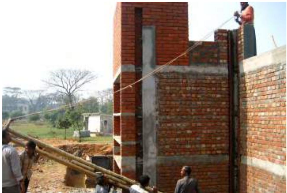
8.78. First column pulled into place
