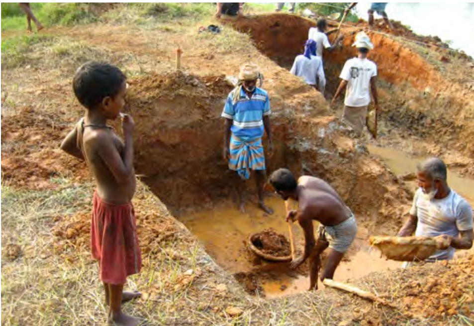
8.15. Workers struggling to pump water out of the excavated area
