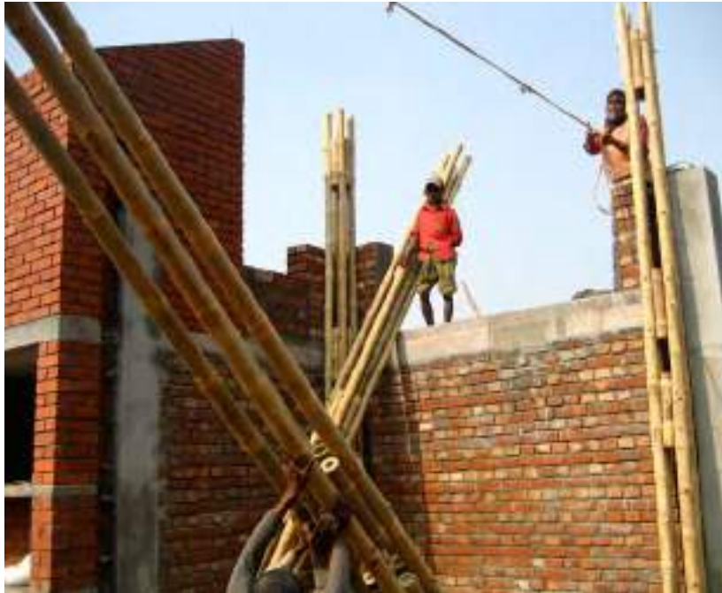
8.79. Bamboo columns carried to position
