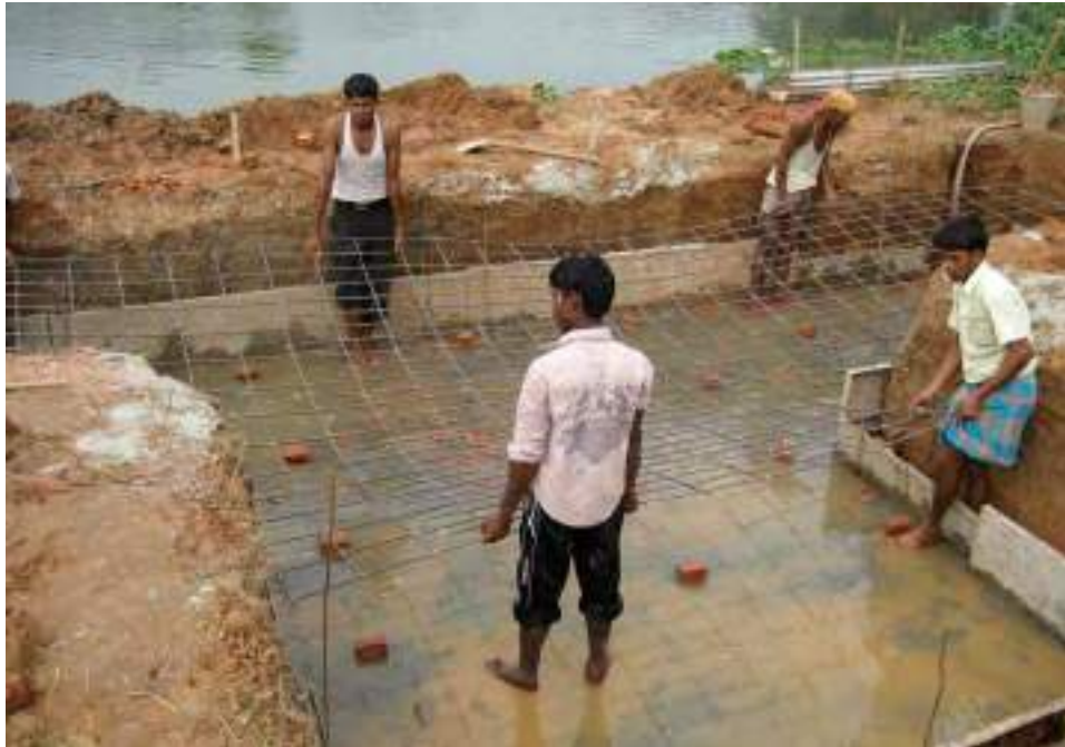
8.24. Reinforcement laid for concrete slab
