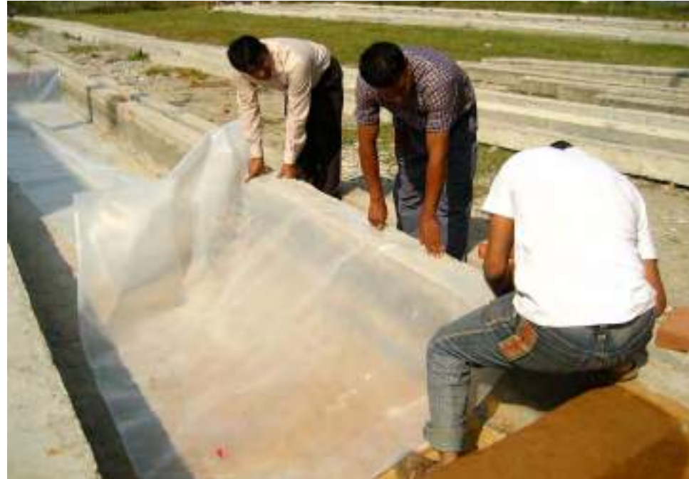
8.33. Preparation of the holding tank for bamboo treatment
