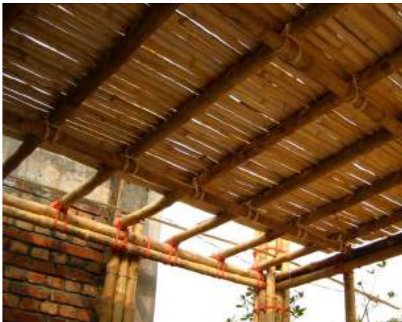
8.97. Underside of second floor
