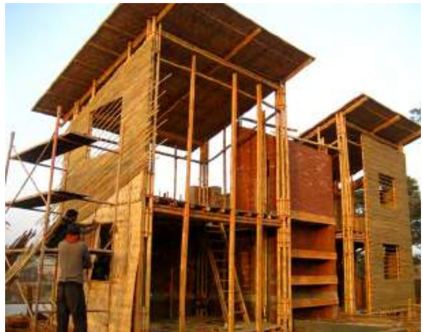
8.137. Installation of side walls
