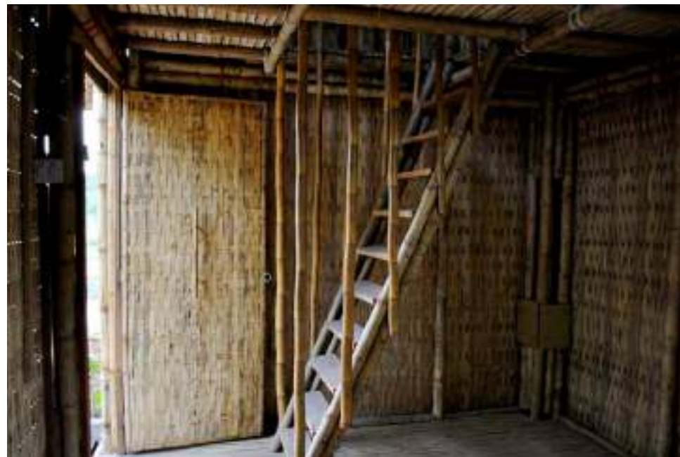
8.134. Interior stairs made of bamboo and wood
