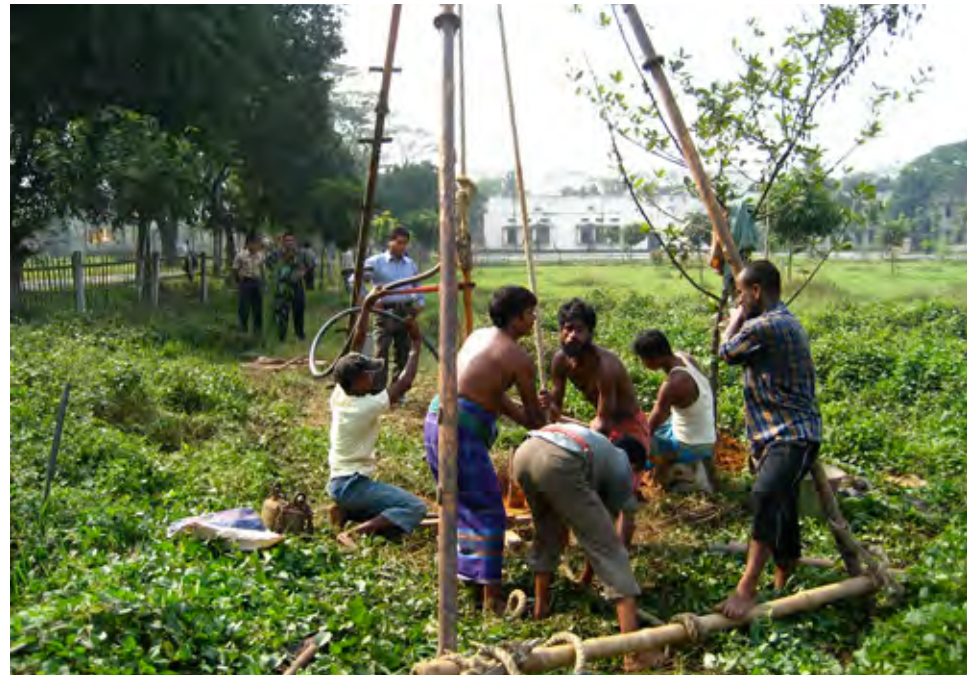
8.0. Soil test conducted on site
