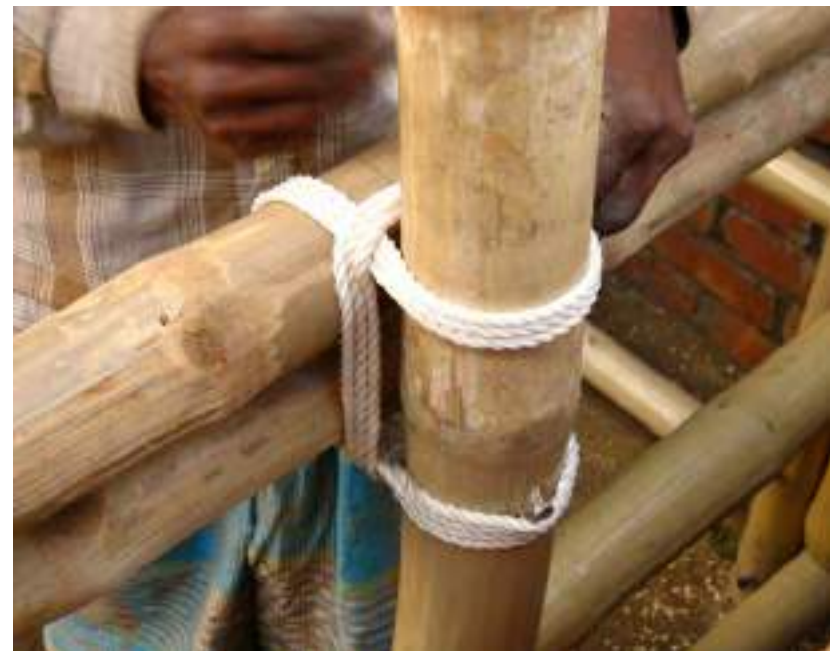
8.82. Nylon tied around bamboo connection
