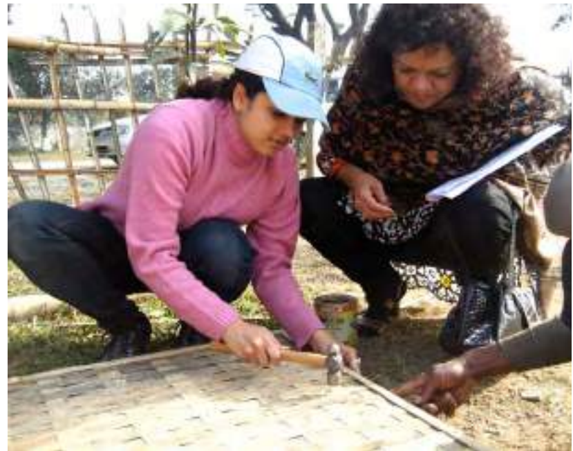
8.143. Wood door frame covered with bamboo cladding
