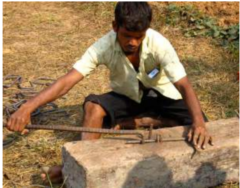
8.48. Worker bending dowels
