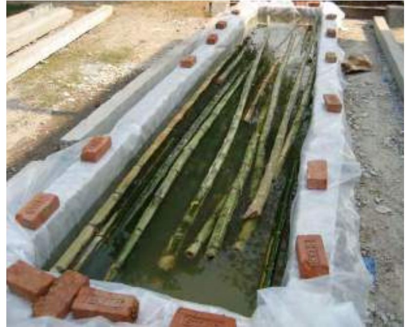
8.47. Chemical treatment of the bamboo before installment
