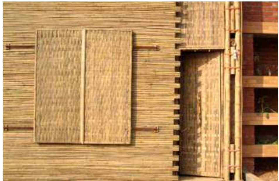
8.153. Application of bamboo in many different finishes
