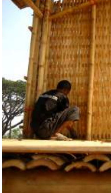
8.118. Installment of walls
