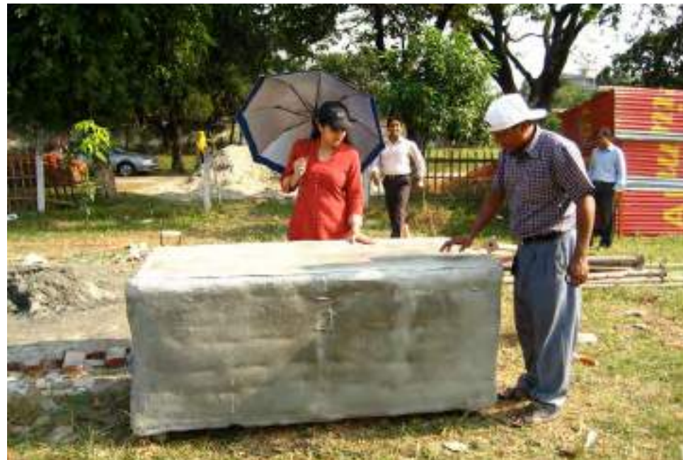
8.40. Inspection of the second foundation model before testing
