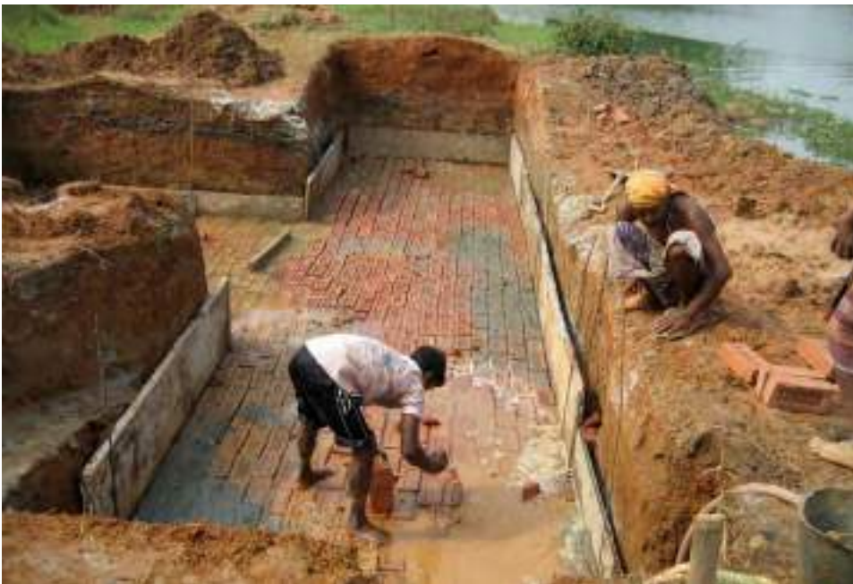
8.21. Brick soiling prepared for concrete slab
