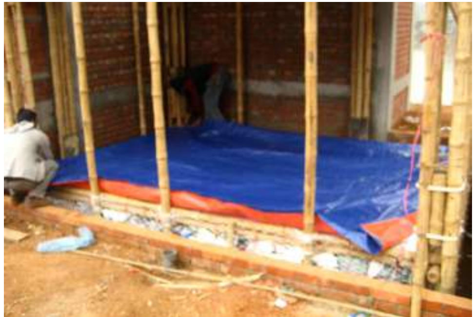
8.109. Water barrier placed on top of water bottle foundation
