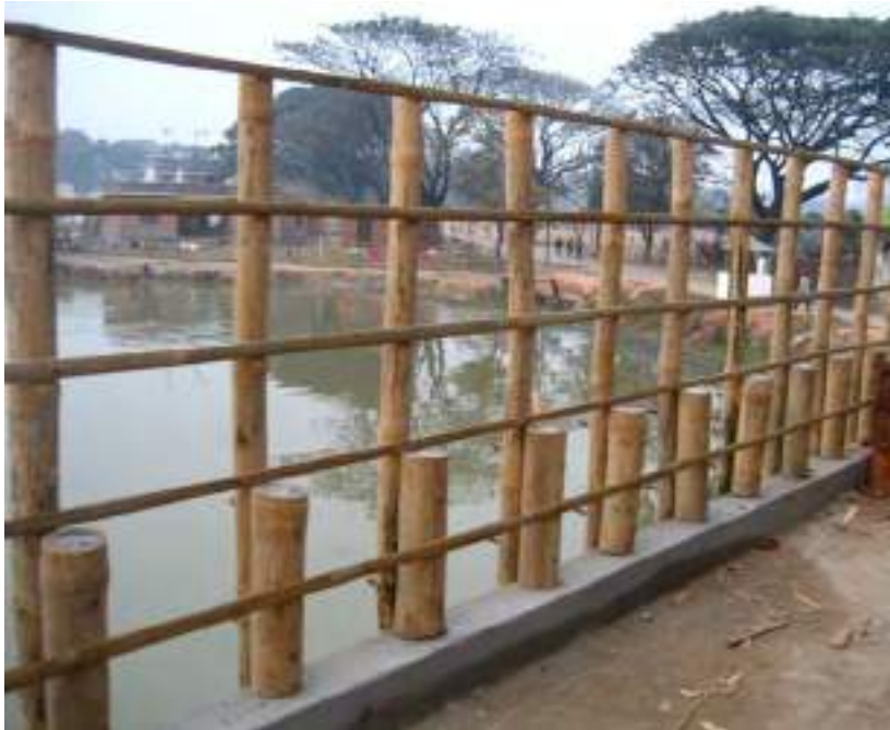
8.129. Finished bamboo railing on top slab of service spine
