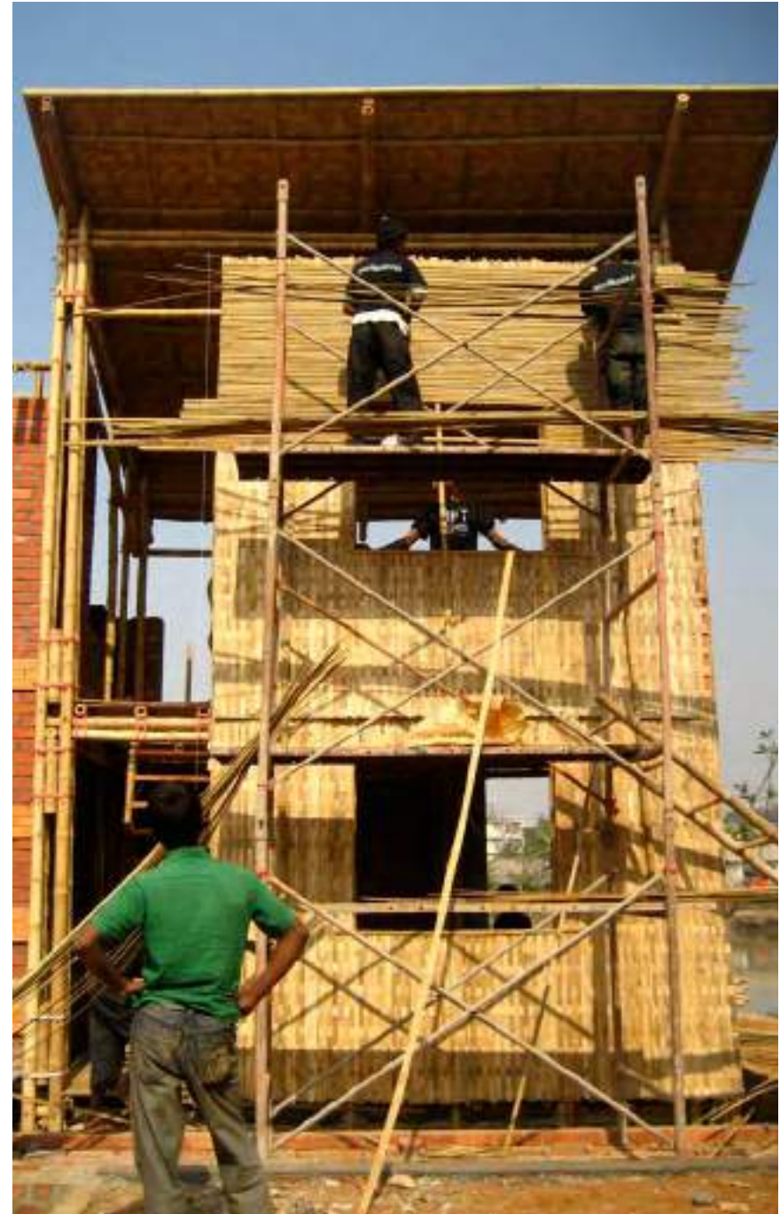
8.126. Installation of front wall finish
