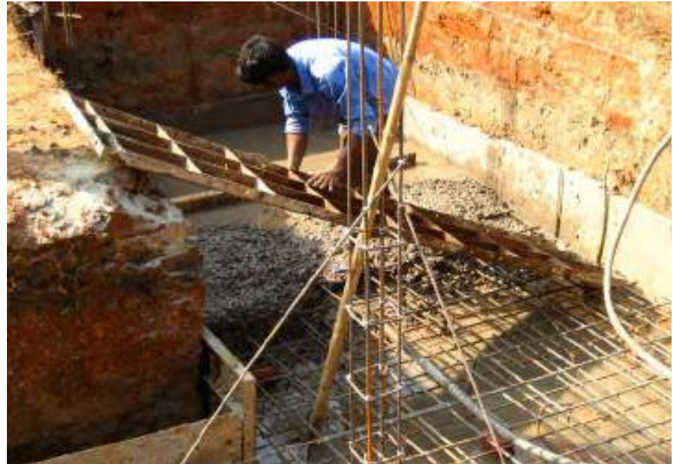
8.27. Worker pouring service spine floor slab
