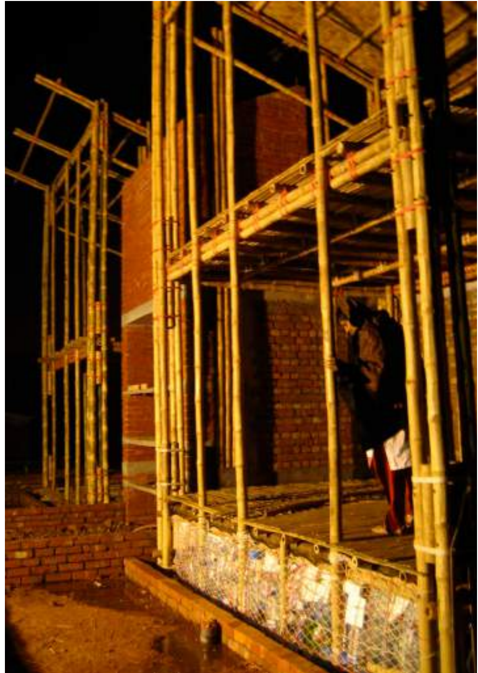
8.111. Water bottle foundation dwelling in buoyant state
