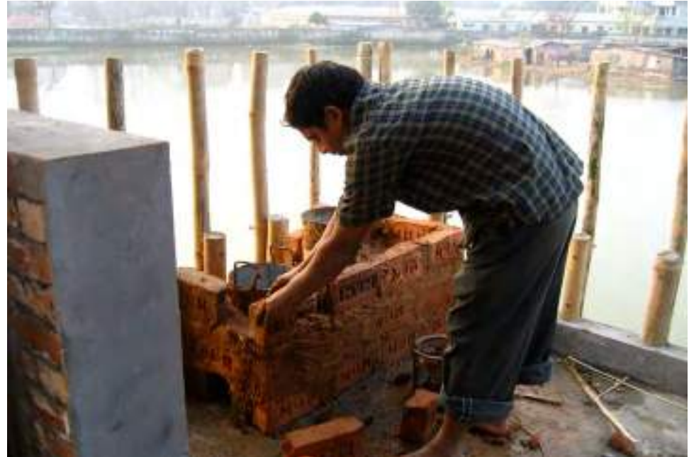
8.128. Installation of Grameen Shakti improved stove
