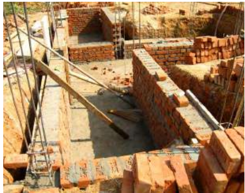
8.32. Service spine walls and columns for water cisterns completed halfway
