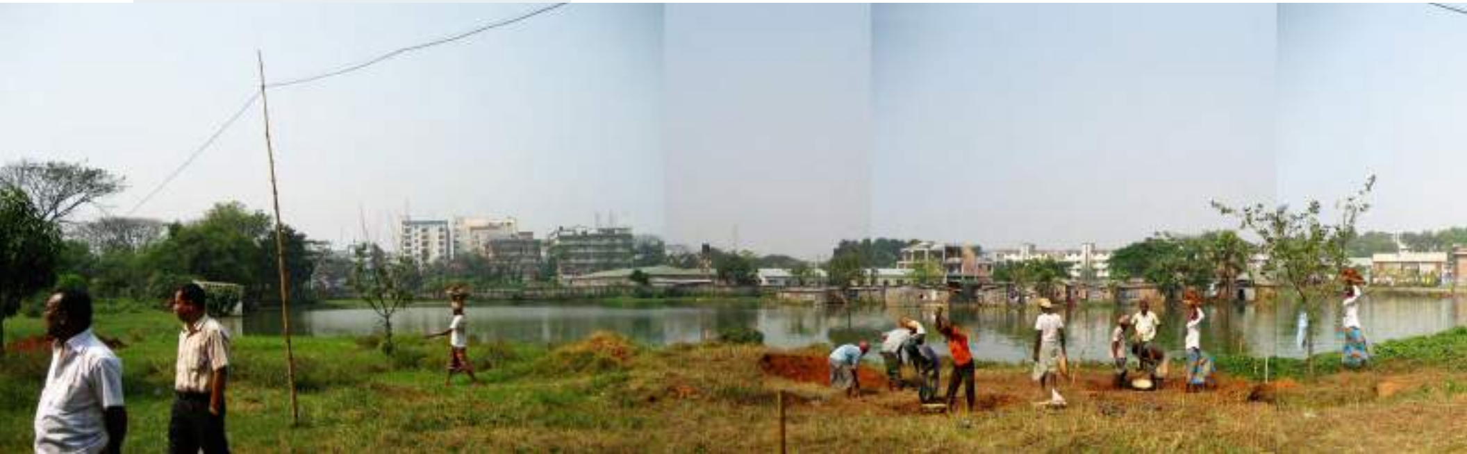
8.16. Workers excavating the site manually
